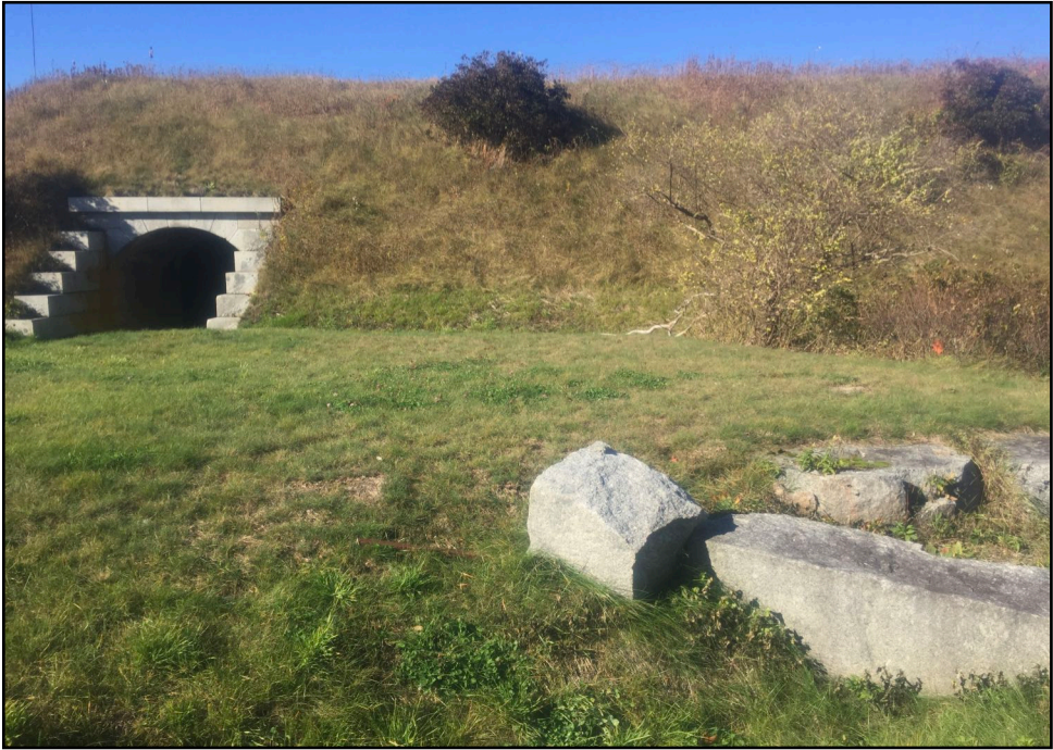
2 SALLY PORT ENTRANCE & EARTHEN BERM Looking west inside the Parade Grounds
