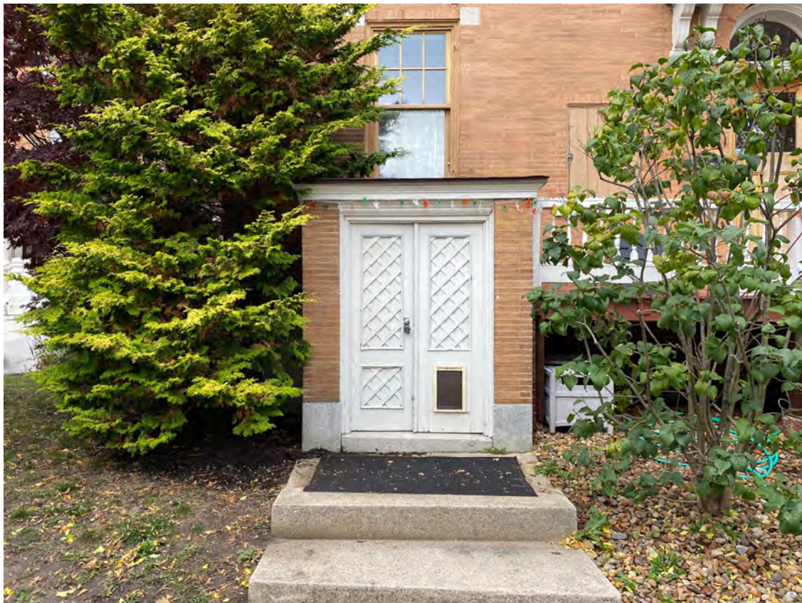
Existing Bulkhead & Exterior Steps
