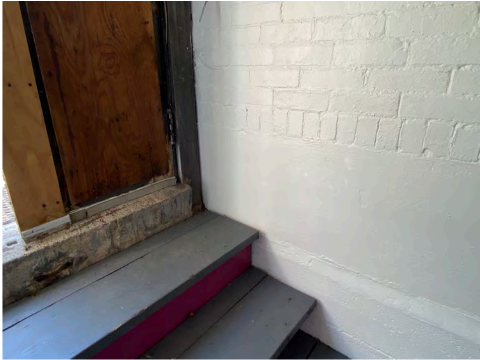
Door condition & transitions from brick to cast stone to foundation
