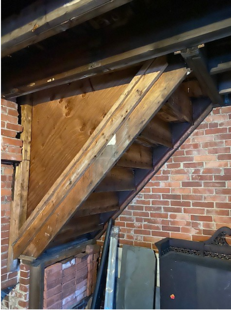
Stair to the former roof deck. Access closed off from the house.
