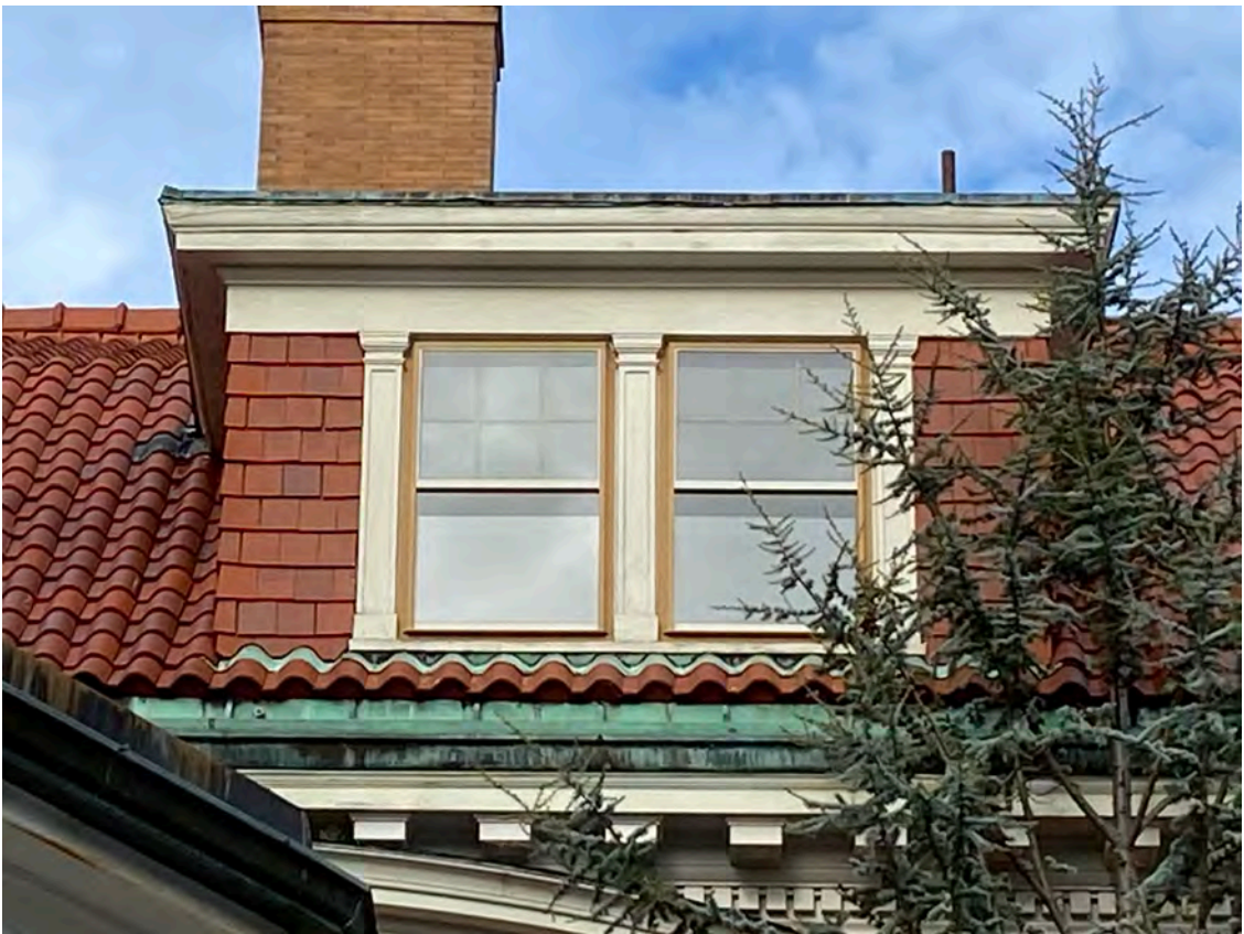
Shed dormer with classical pilasters as window trim
