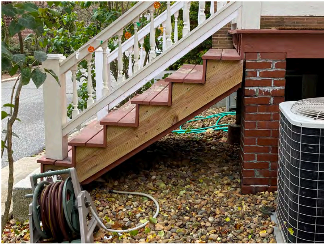
Existing stair risers range from 6-1/2" to 8-1/2" and pitch downward
