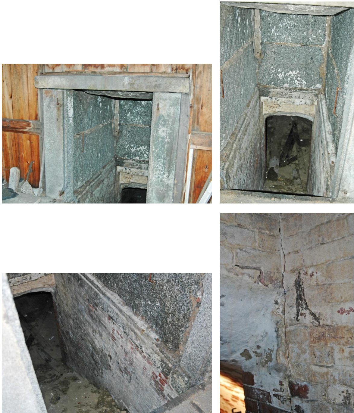
Figure 62. City tomb entrance. Upper left shows the entrance to the tomb stairs from the “Dead House.” Note the pintles for a set of vertical doors on the granite supports on each side of the entrance. Upper right shows the above grade granite structure and at the base of the stairway, the entrance into the tomb. Lower left shows the right (north) sidewall of the entrance. The stairs are no longer in place. In their place is a ramp of sand. The lower right photo shows a stress crack in the brick corners under the above grade granite west wall.
