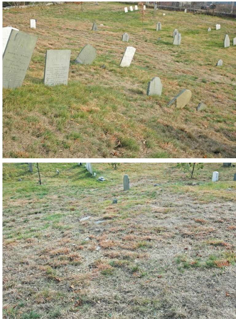
Figure 78. Erosion at the eastern slope in the cemetery. The upper photograph shows how this erosion has caused stones in this area to lean – these should be reset. The lower photograph illustrates compaction on this slope that is causing rainwater to run off, rather than be absorbed.
