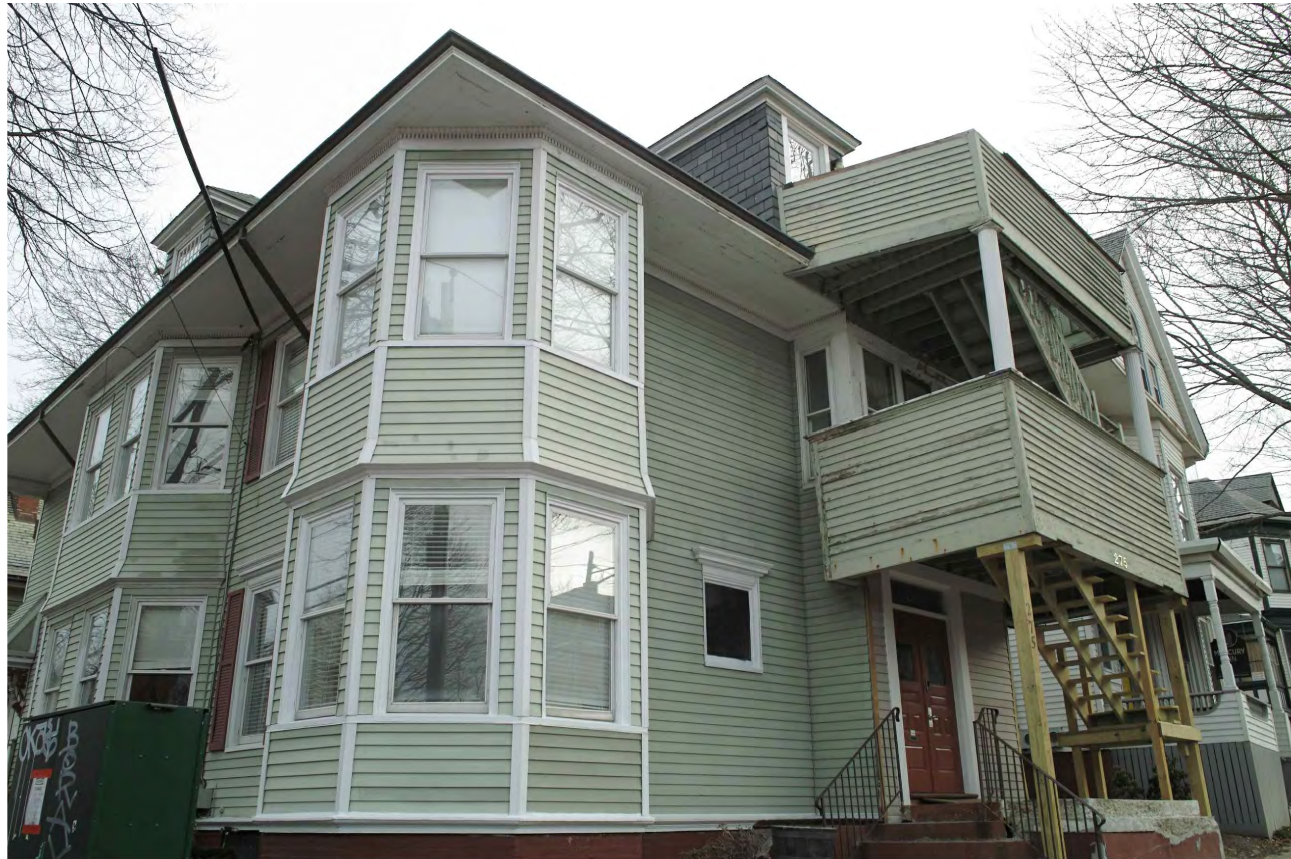
1 WEST FACADE FROM NORTHWEST
