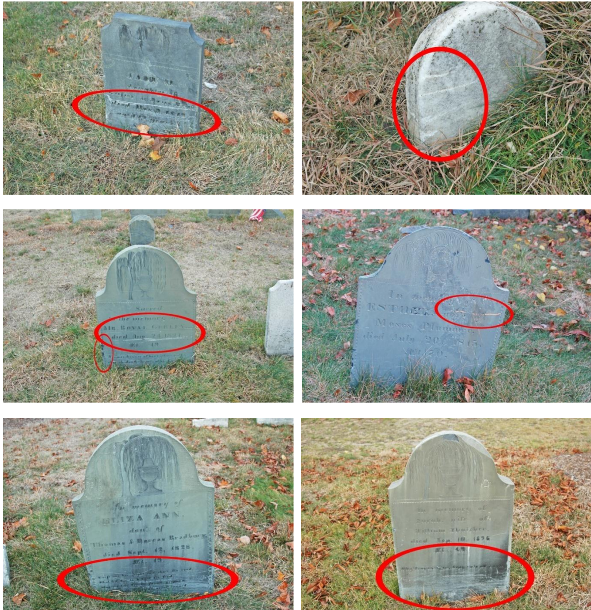
Figure 71. Examples of mower and trimmer damage to stones in Eastern Cemetery. Upper and middle photos show typical scrapes and damage caused by mowers. The photo on the middle right reveals paint transfer from the mower onto the stone itself. The photos in the bottom row show parallel striations on the stones caused by careless trimmer use with a line too heavy for cemetery work.
