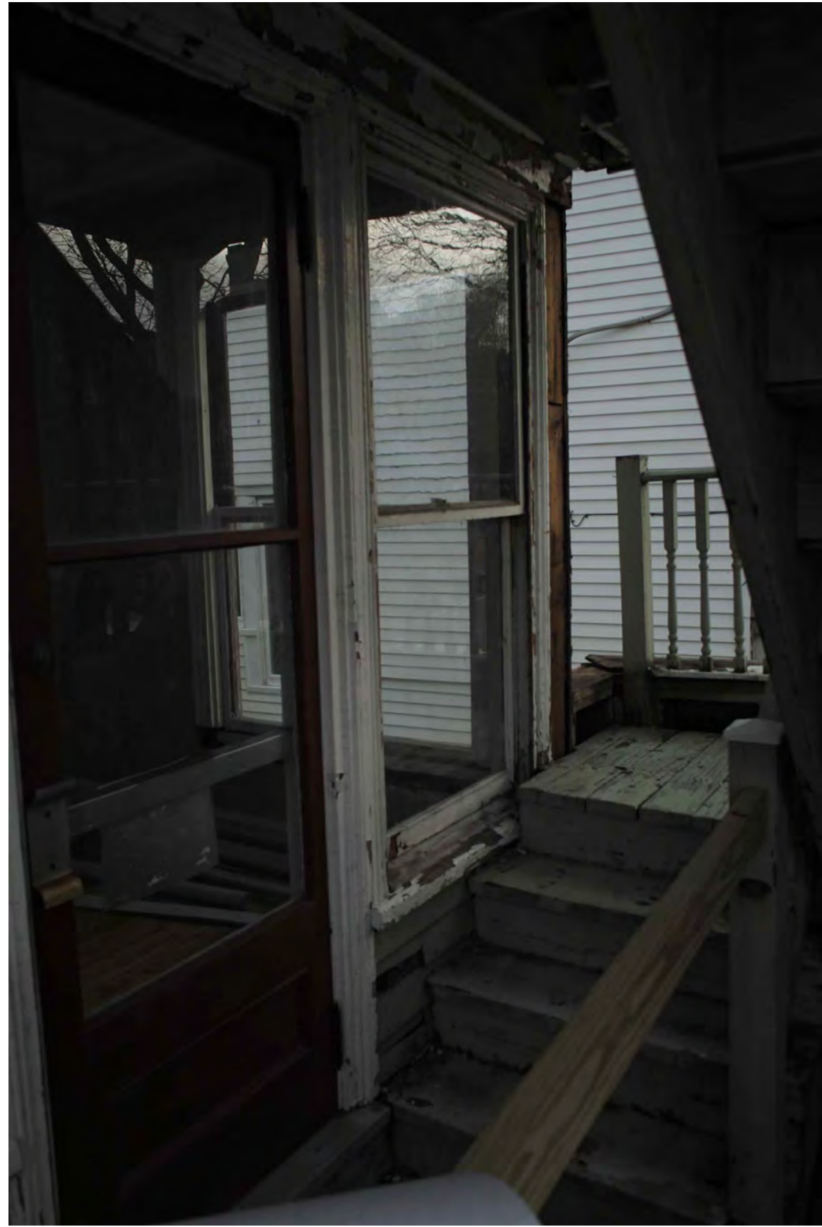
1 DOOR AND WINDOW AT SECOND FLOOR DECK
