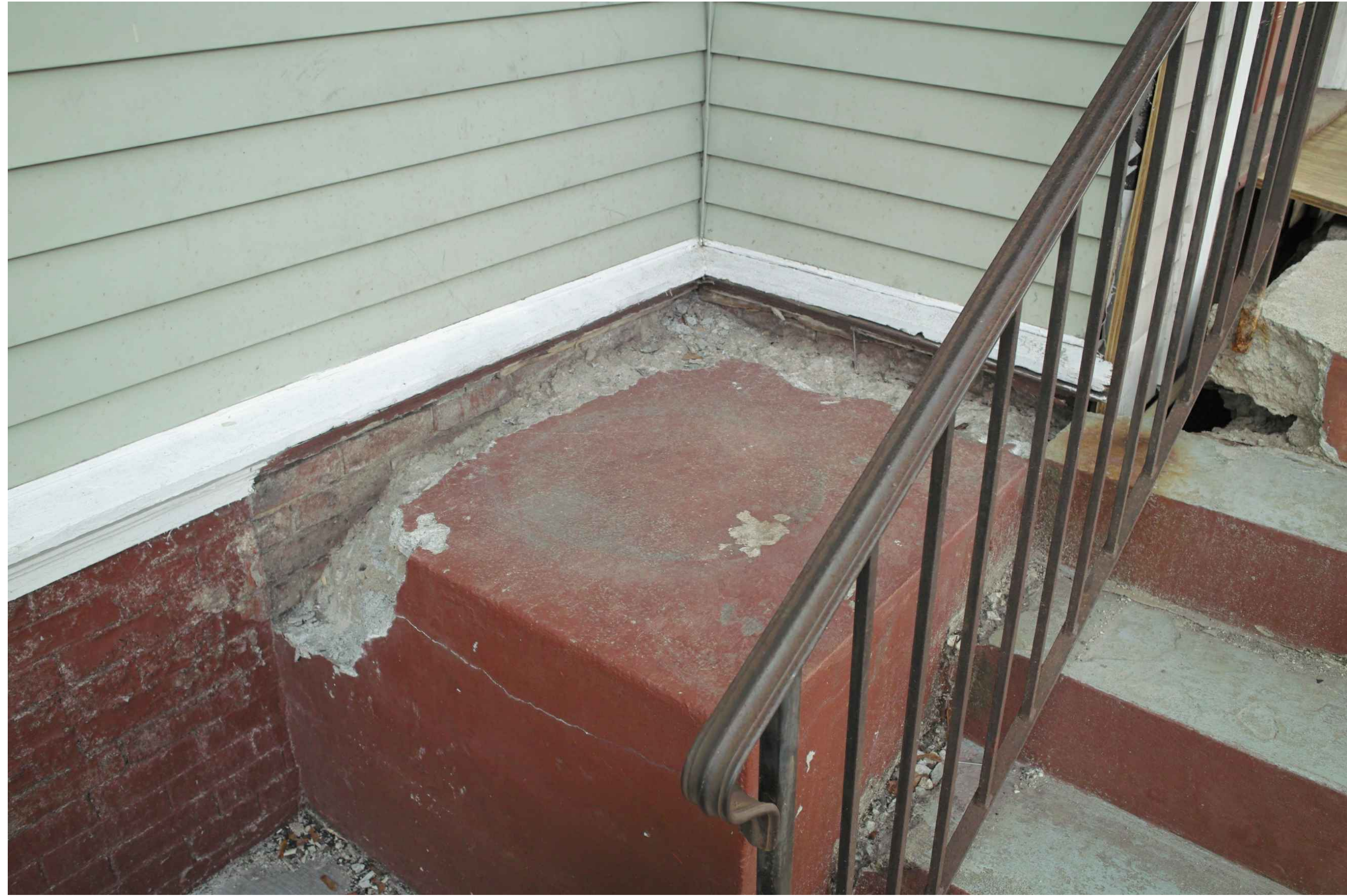
4 CONDITION AT EXISTING STAIR AND PORCH
