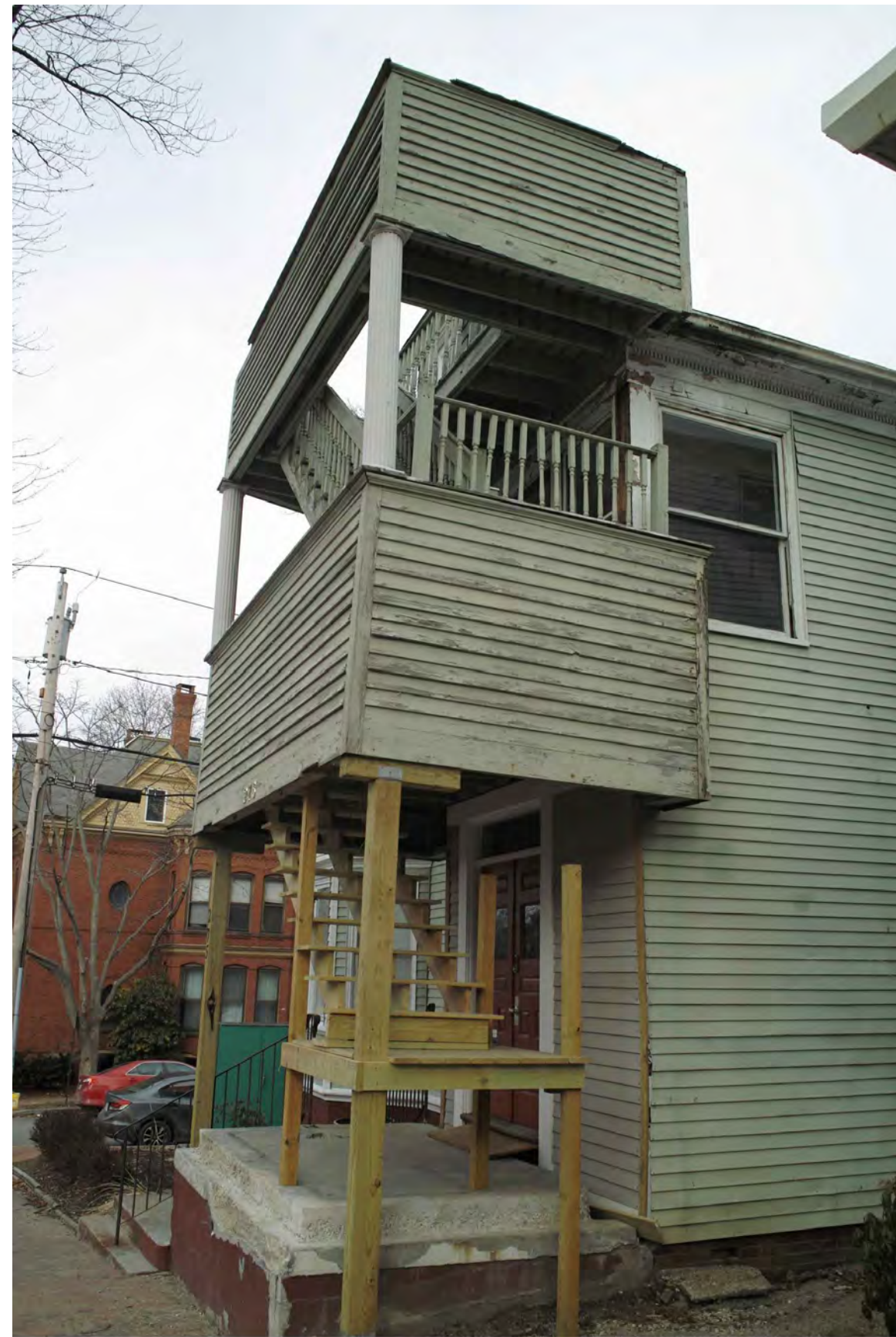
1 WEST FACADE FROM SOUTHWEST
