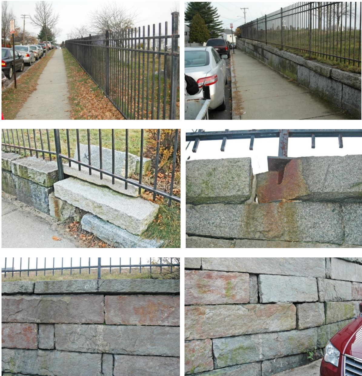
Figure 58. Mountfort Street fence and wall. Upper left photo shows the fence, looking to the northeast. Upper right shows the fence set on the granite retaining wall. Middle left shows where the granite wall has been “extended” by dumping granite coping. Middle right photo shows where iron jacking has split the granite coping. Lower left photo shows loss of mortar in the joints of the wall. Note also the crack that has formed from iron jacking at the line post in the center of the photo. Lower right shows a noticeable bulge in the wall on Mountfort. Joints are open and the retaining rock is set back in the wall, showing the movement outward.
