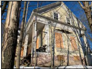
② BACK PORCH WITH STACK OF INTERIOR TRIM THAT WILL BE USED AS TEMPLATES FOR REHABILITATION
