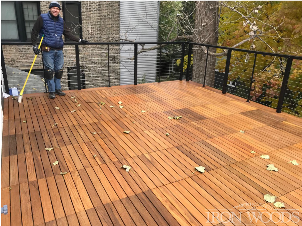
ROOF TOP DECK TILES
