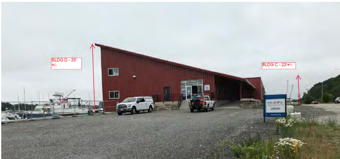
Existing Buildings C and D
