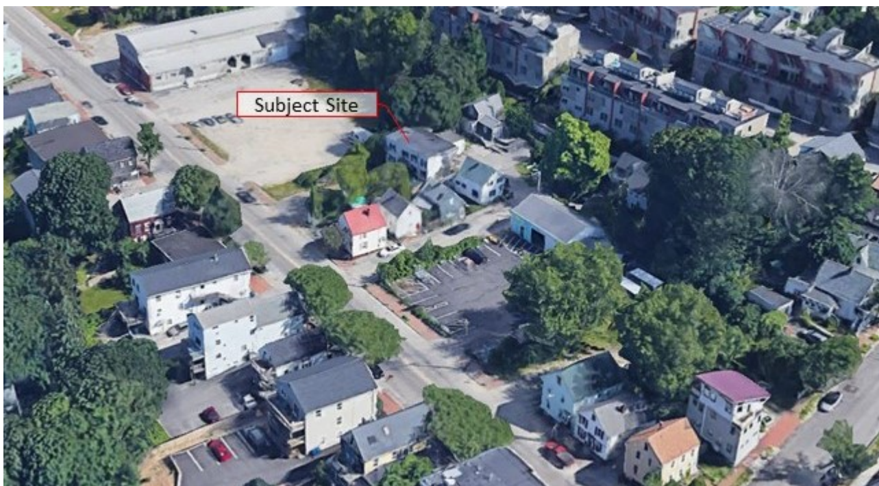
Aerial view of 163 Washington Avenue
