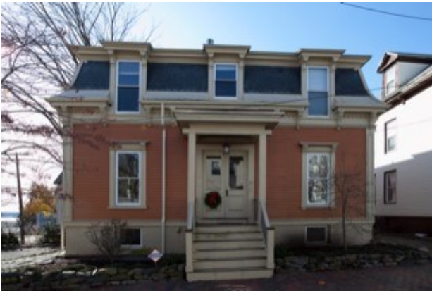
The Second Empire at 60 Kellogg Street retains its historic slate roof, window hoods, and corner boards.
