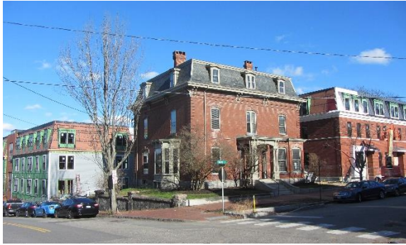
Affordable housing projects under construction on Deering & Cumberland
