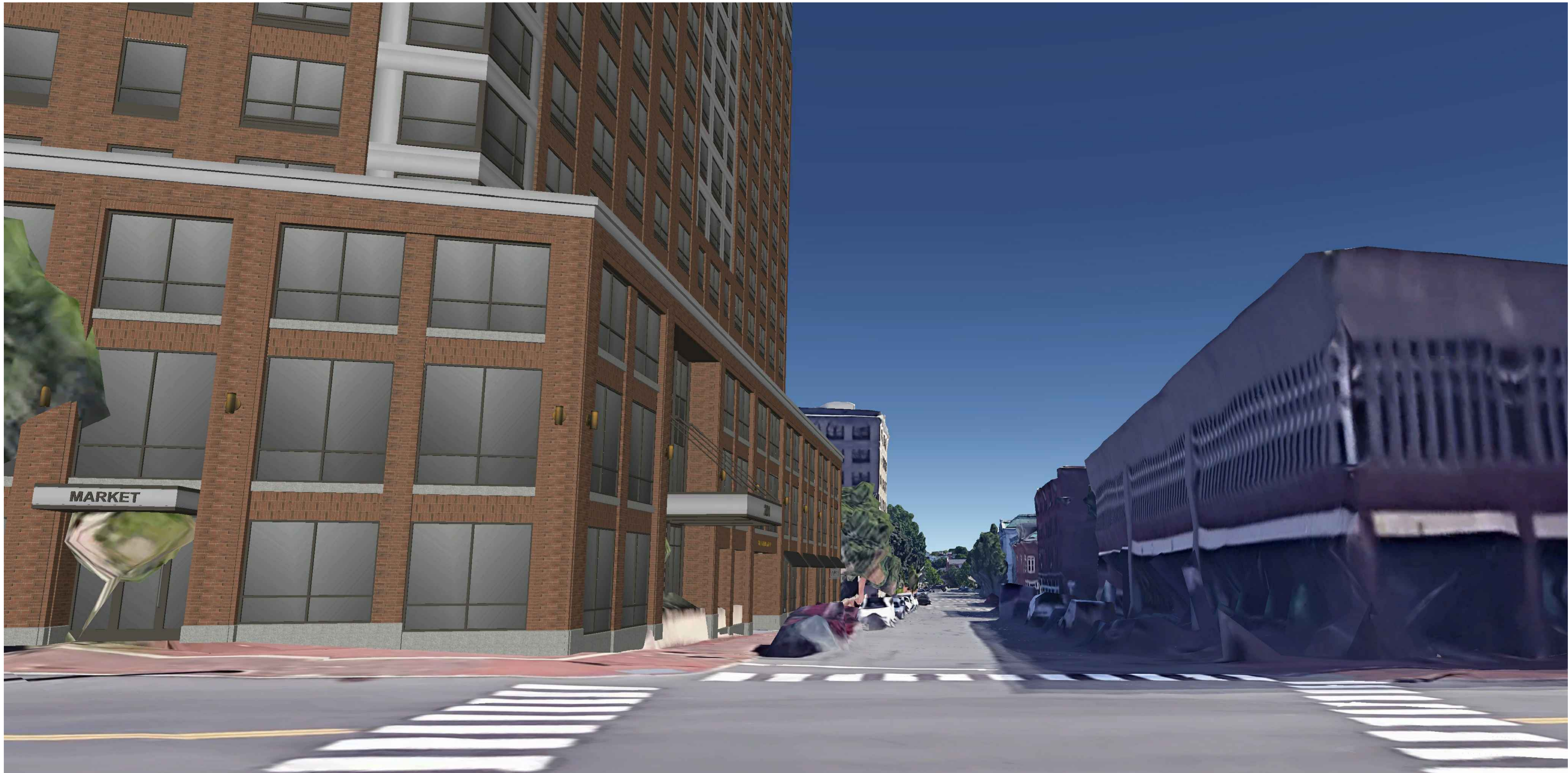
VIEW LOOKING EAST FROM FEDERAL STREET
