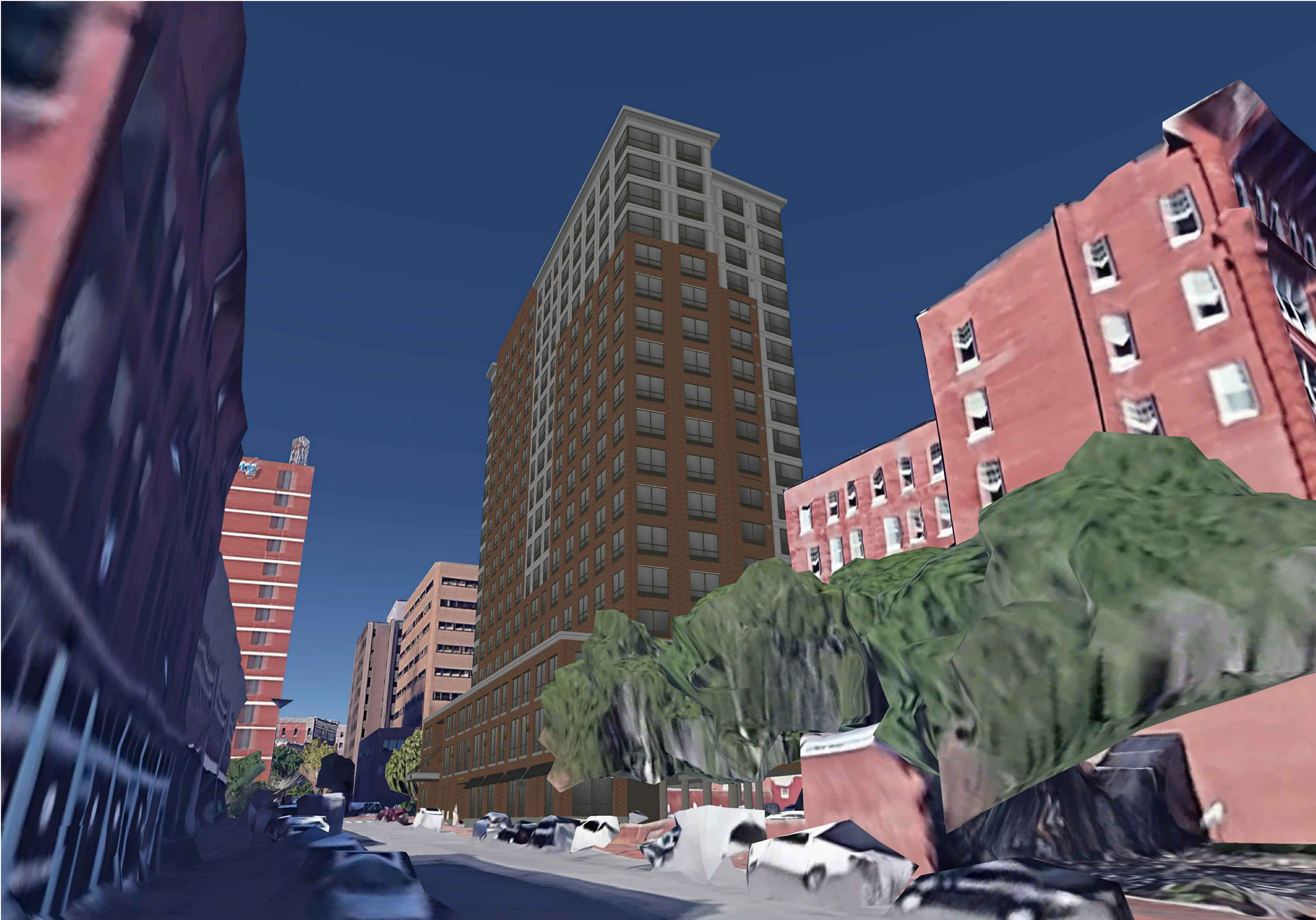
VIEW LOOKING WEST FROM EXCHANGE STREET
