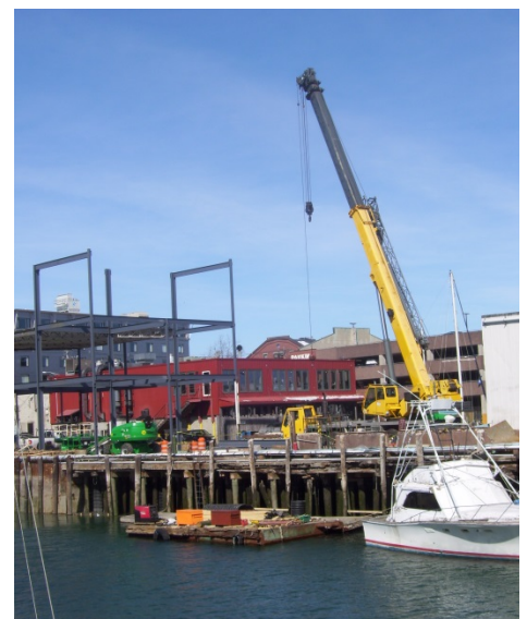
Development of the “Scales” building on Maine Wharf, 2014. Subject to the 55% rule
