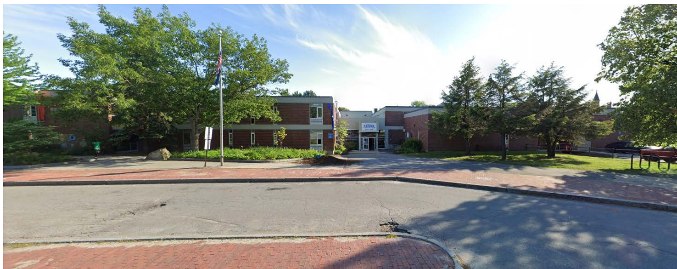
Figure 3: Existing Conditions (Image from Front of Reiche Elementary School) – Source: Google Earth
