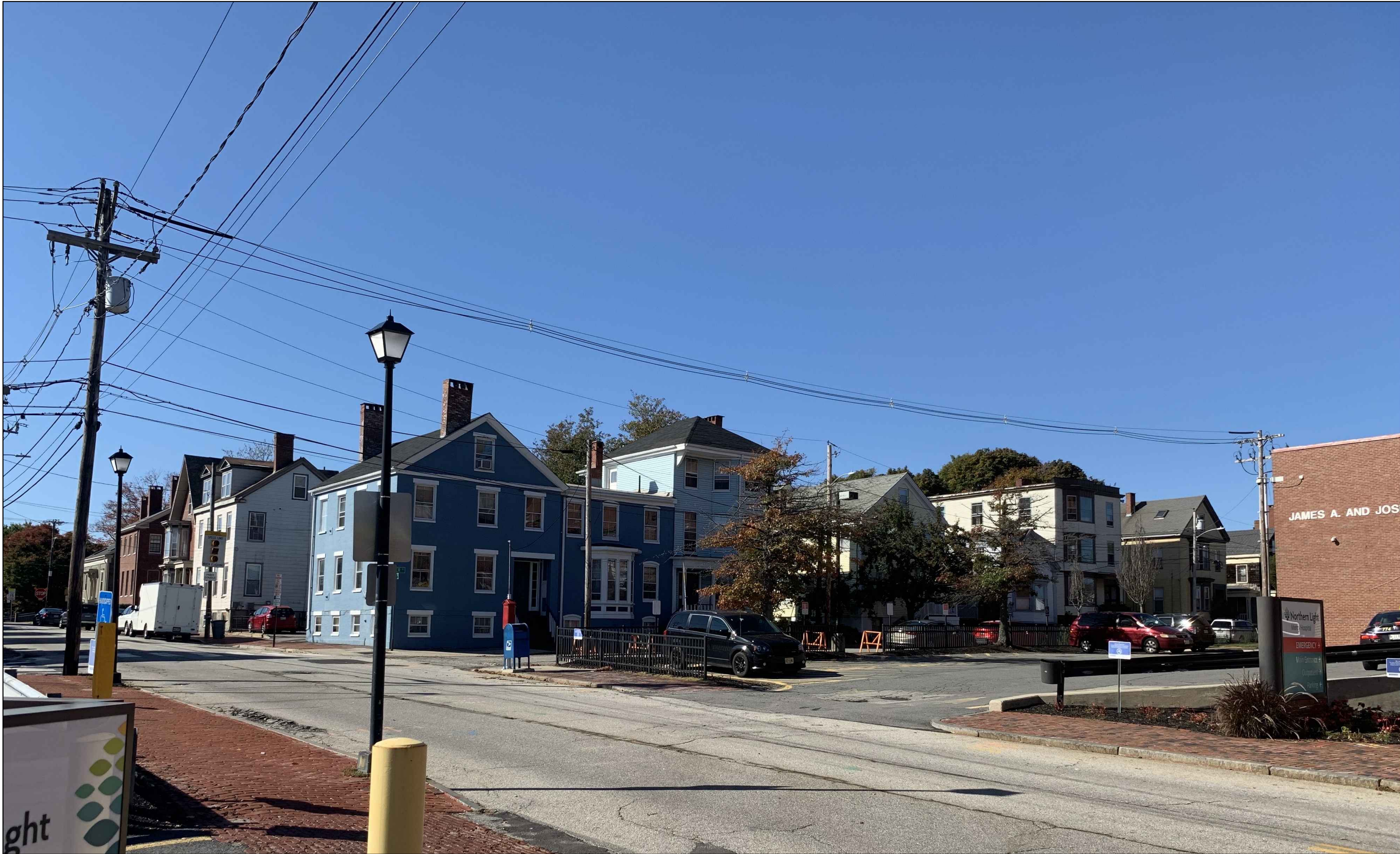
1 VIEW LOOKING SOUTH ON SPRING STREET - EXISTING
