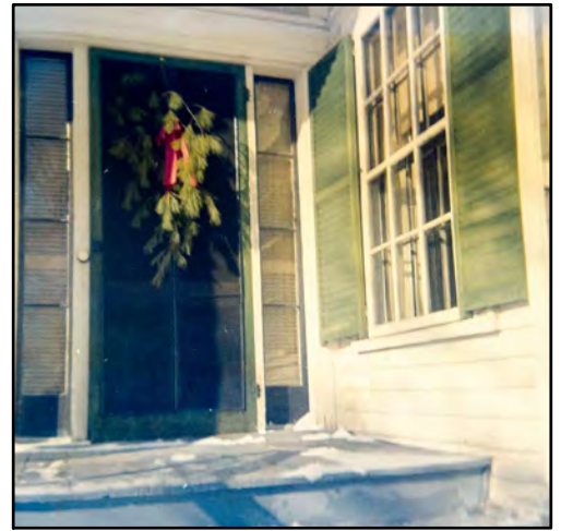
② ORIGINAL SIDE LIGHTS AT FRONT DOORS
