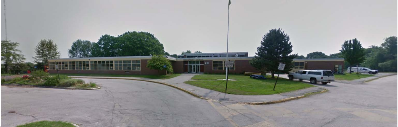
Figure 3: Existing Conditions (Image from Building Front) Source: Google
