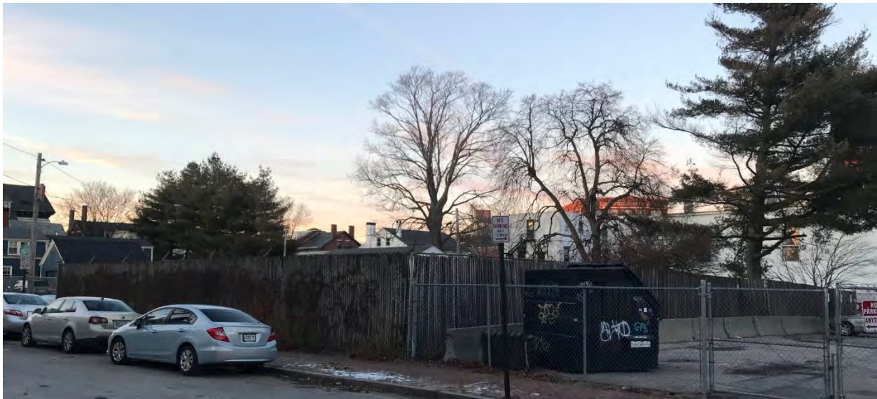
99 Winter Street Existing conditions
