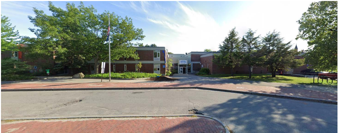
Figure 3: Existing Conditions (Image from Front of Reiche Elementary School) – Source: Google Earth
