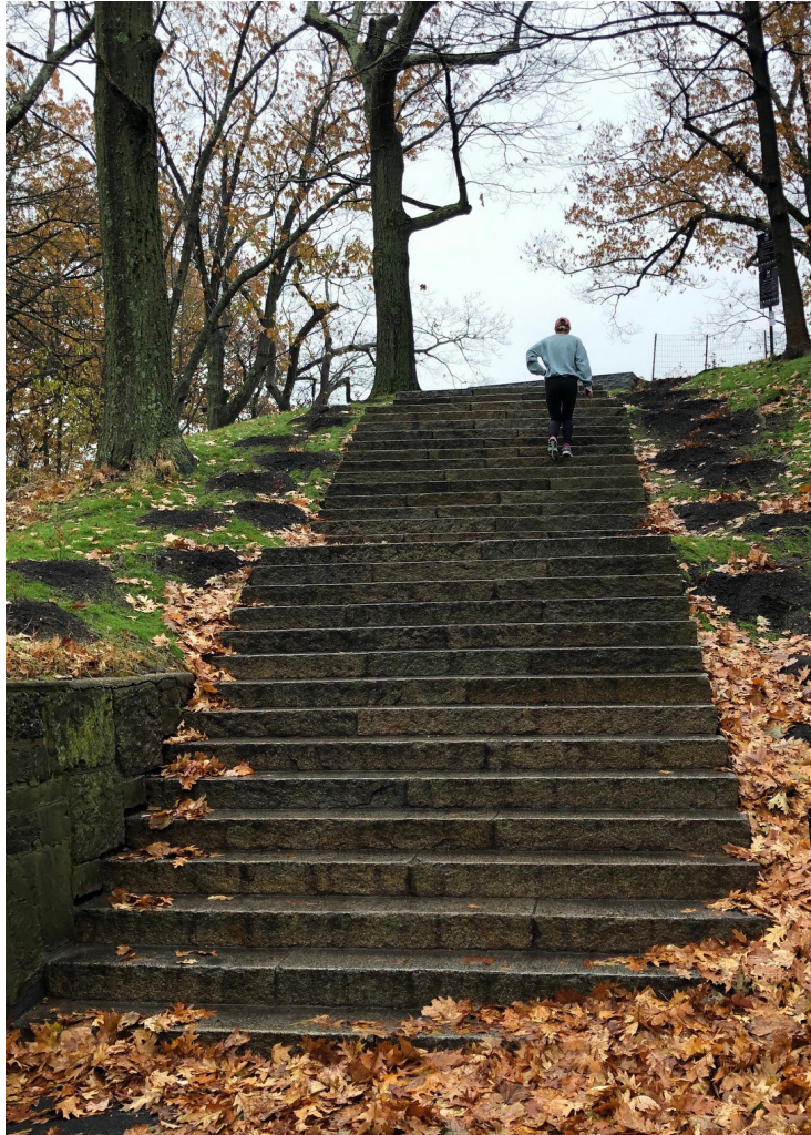
(left) An example of semi-formal granite stairs at a park entry in a historic park. For the stairs at the Valley Street entrance to Western Promenade, the stairs should have handrails that meet International Building Code and ADA Accessibility Guidelines. (Jamaica Pond Park, Boston)
