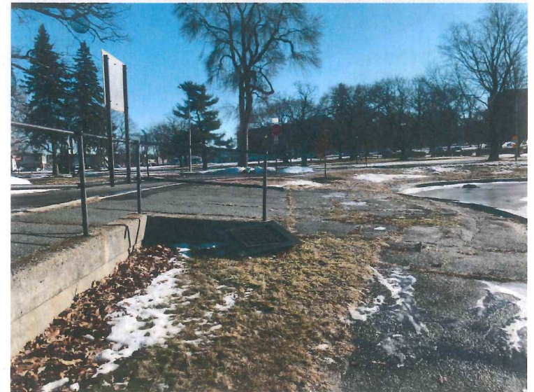
View of existing retaining wall and railing, and location for proposed boat dock
