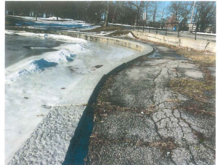
View of existing pond edge and retaining wall with railing.
