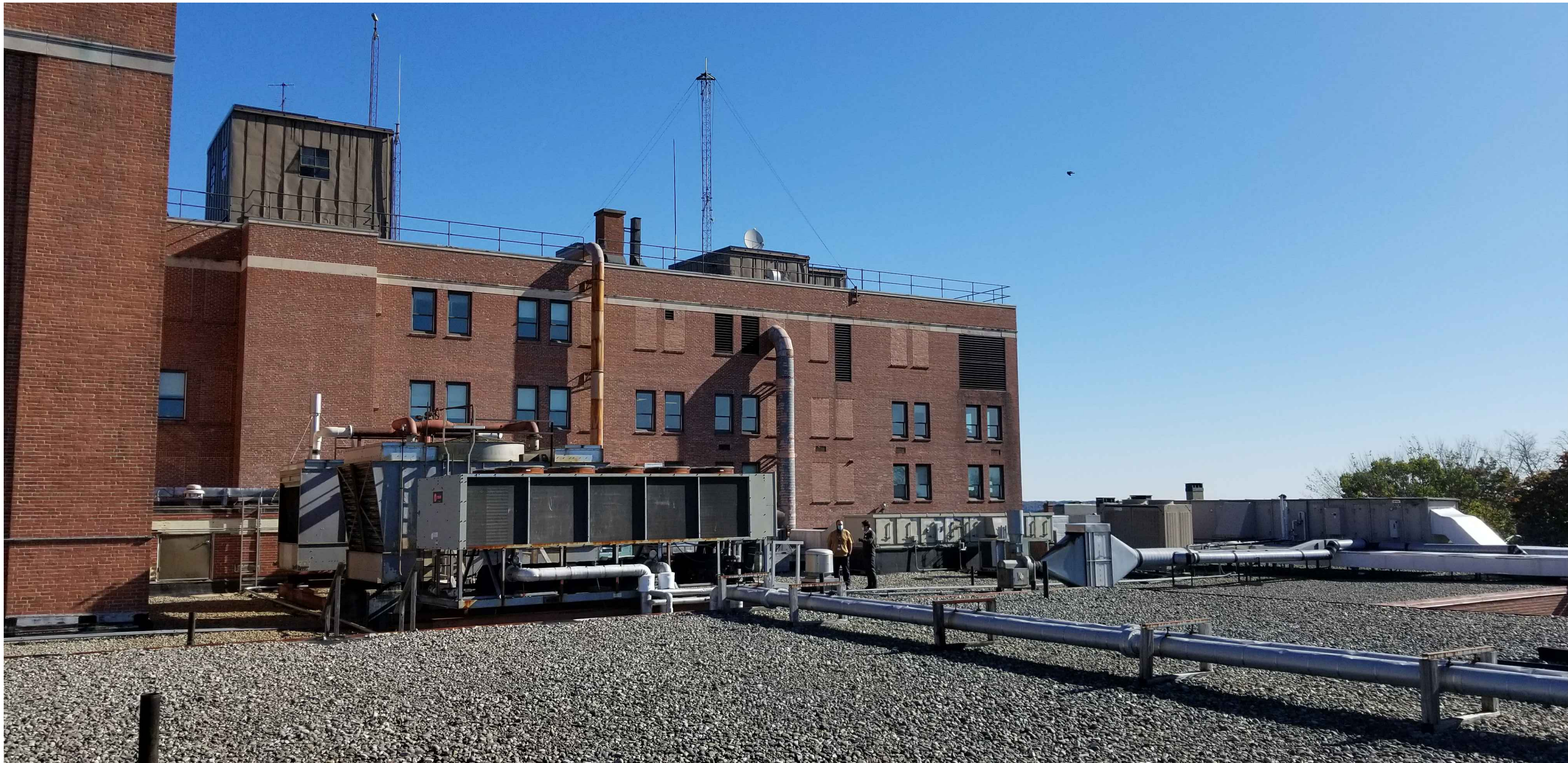
4 VIEW LOOKING NORTH EAST FROM EMERGENCY ROOM ROOF KTS
