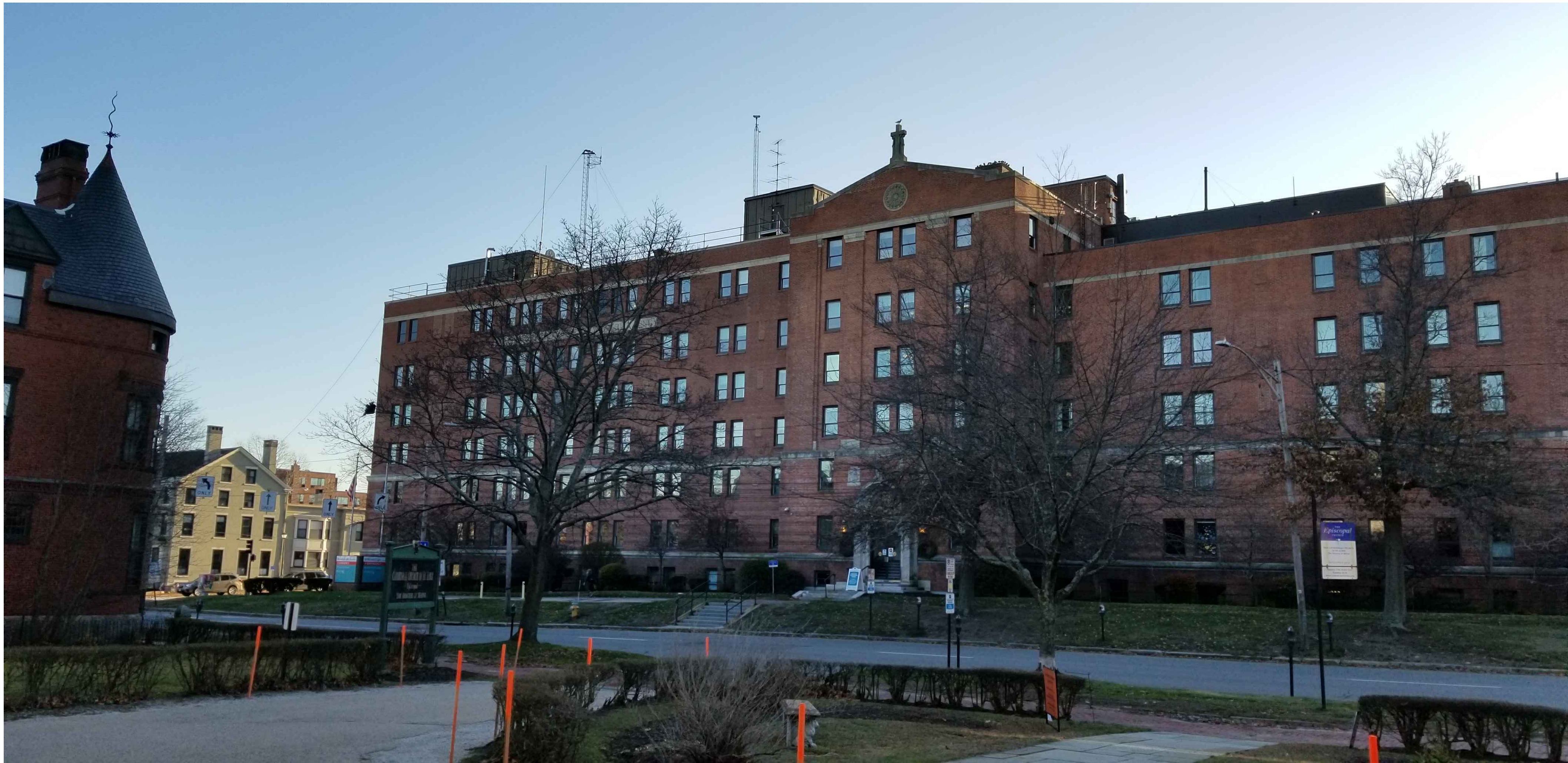
3 VIEW LOOKING SOUTH FROM ST. LUKE'S CATHEDRAL KTS
