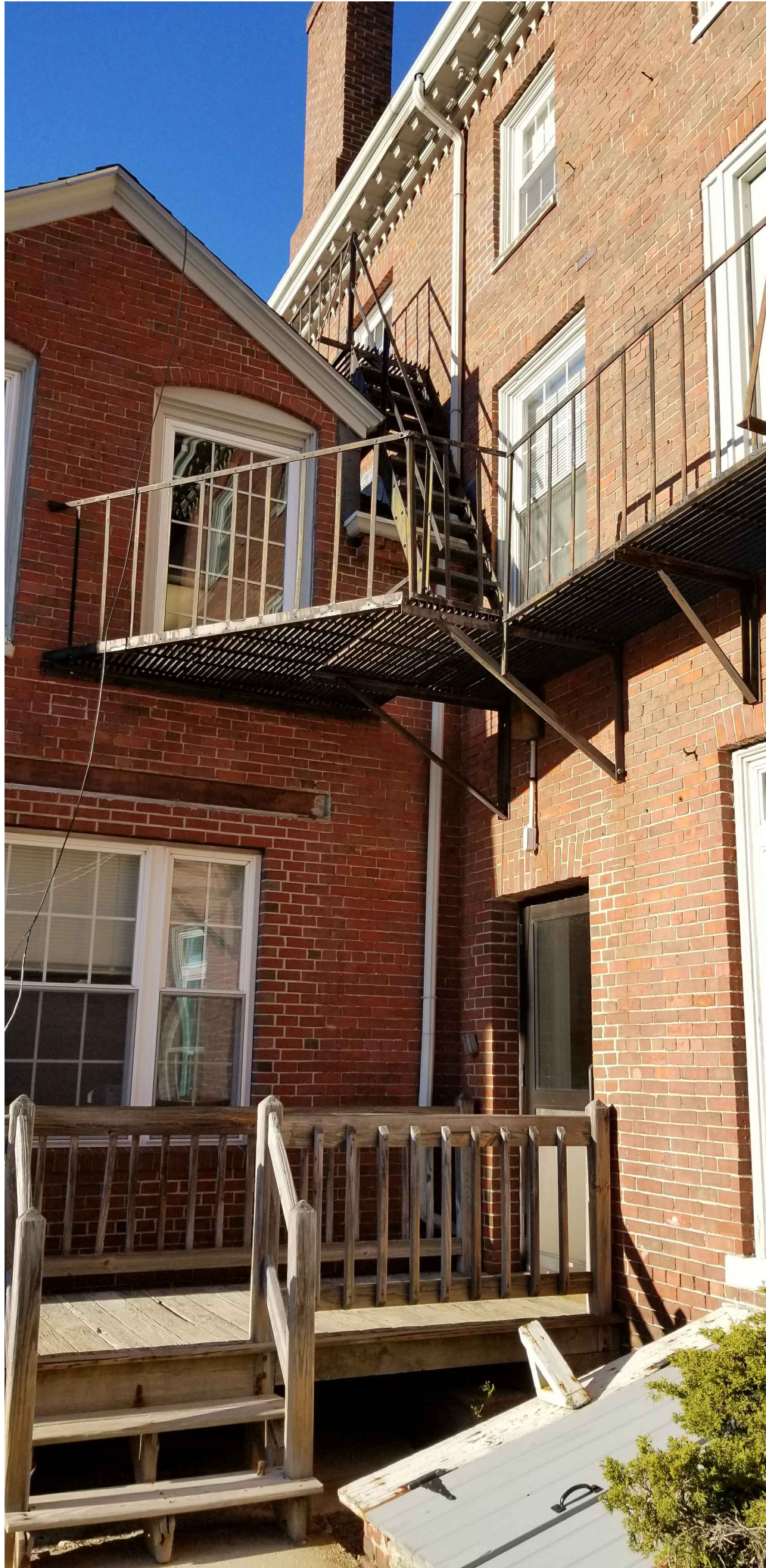
1 VIEW FROM PATIO LOOKING NORTH WEST - EXISTING CONDITIONS
