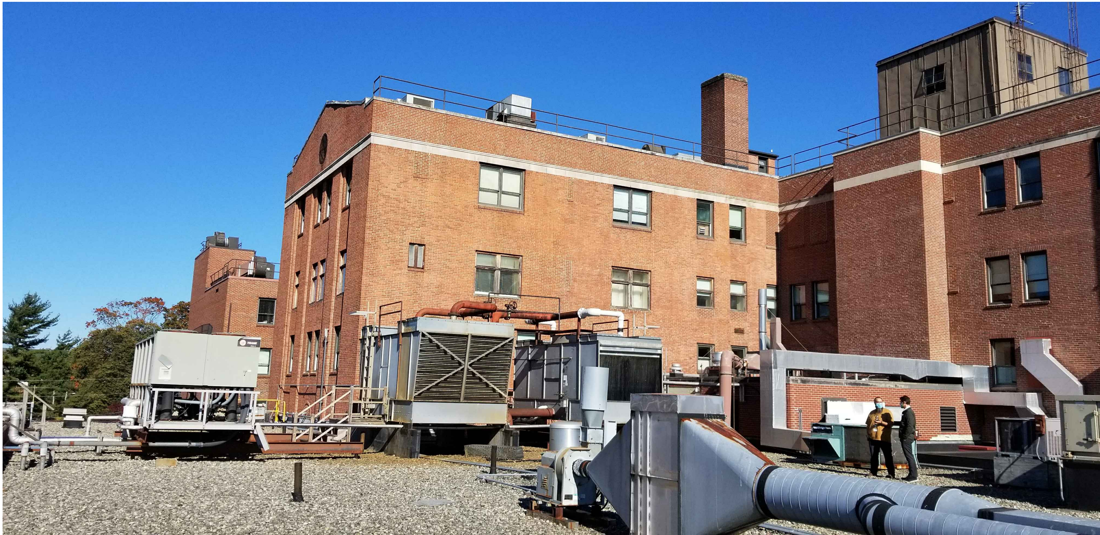
3 VIEW LOOKING NORTH FROM EMERGENCY ROOM ROOF KTS
