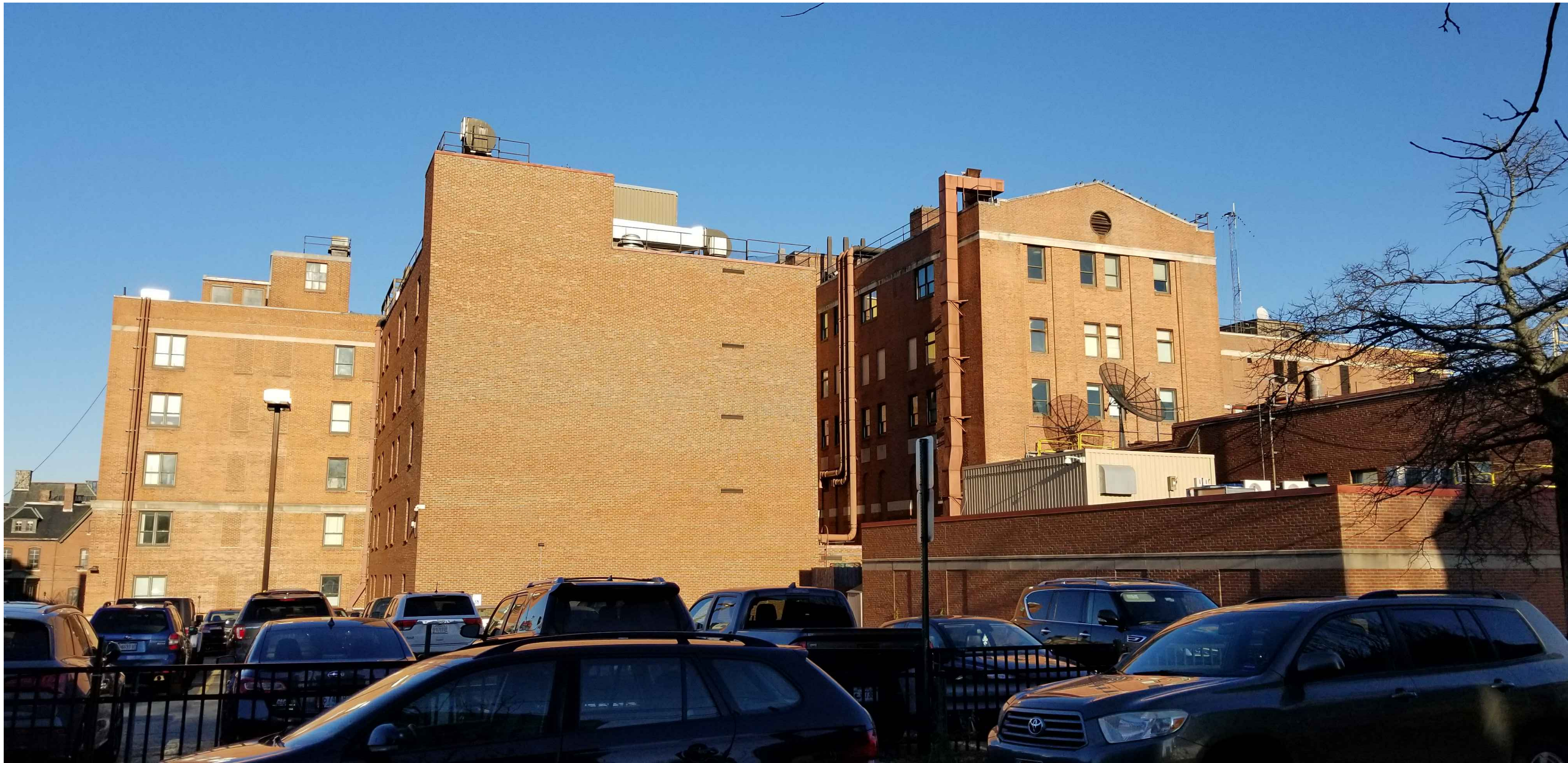
3 VIEW LOOKING NORTH EAST FROM WINTER ST.
