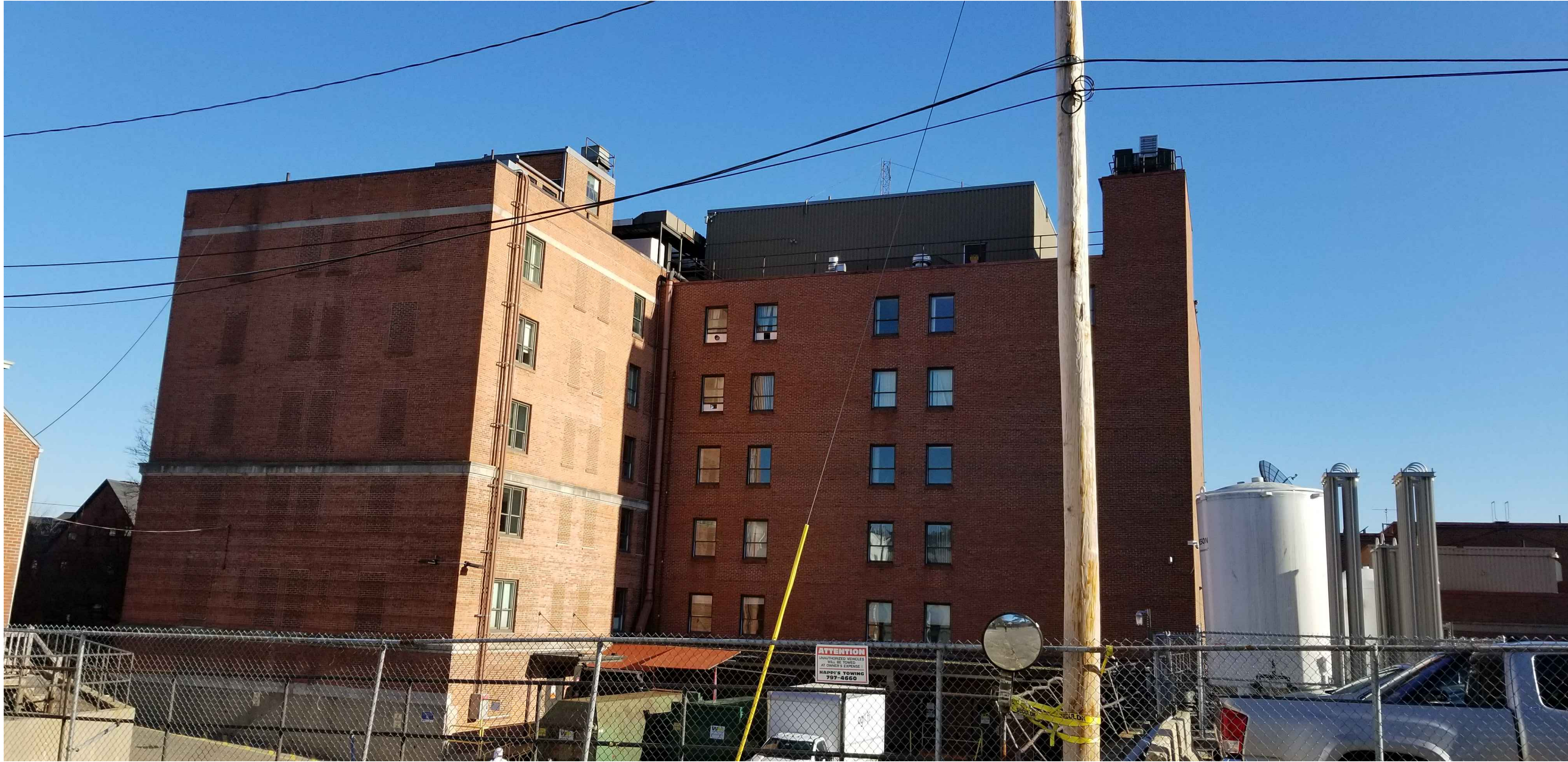
2 VIEW LOOKING EAST FROM THE PORTLAND CLUB KTS
