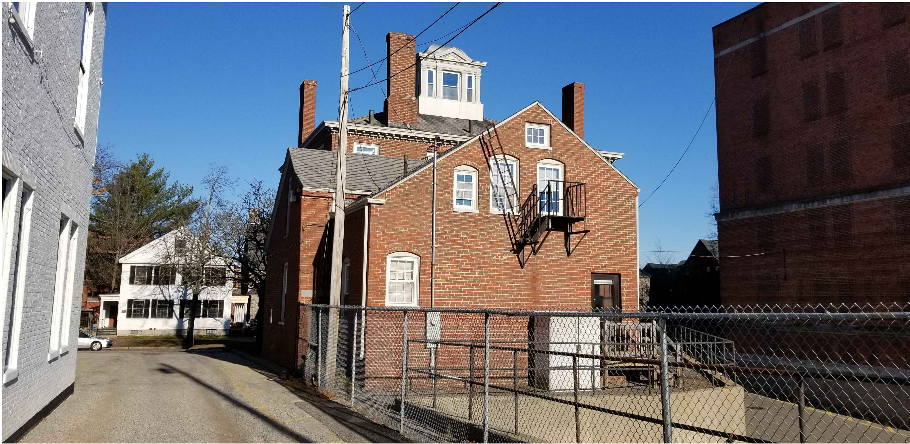
1 VIEW LOOKING NORTH EAST - EXISTING CONDITIONS
