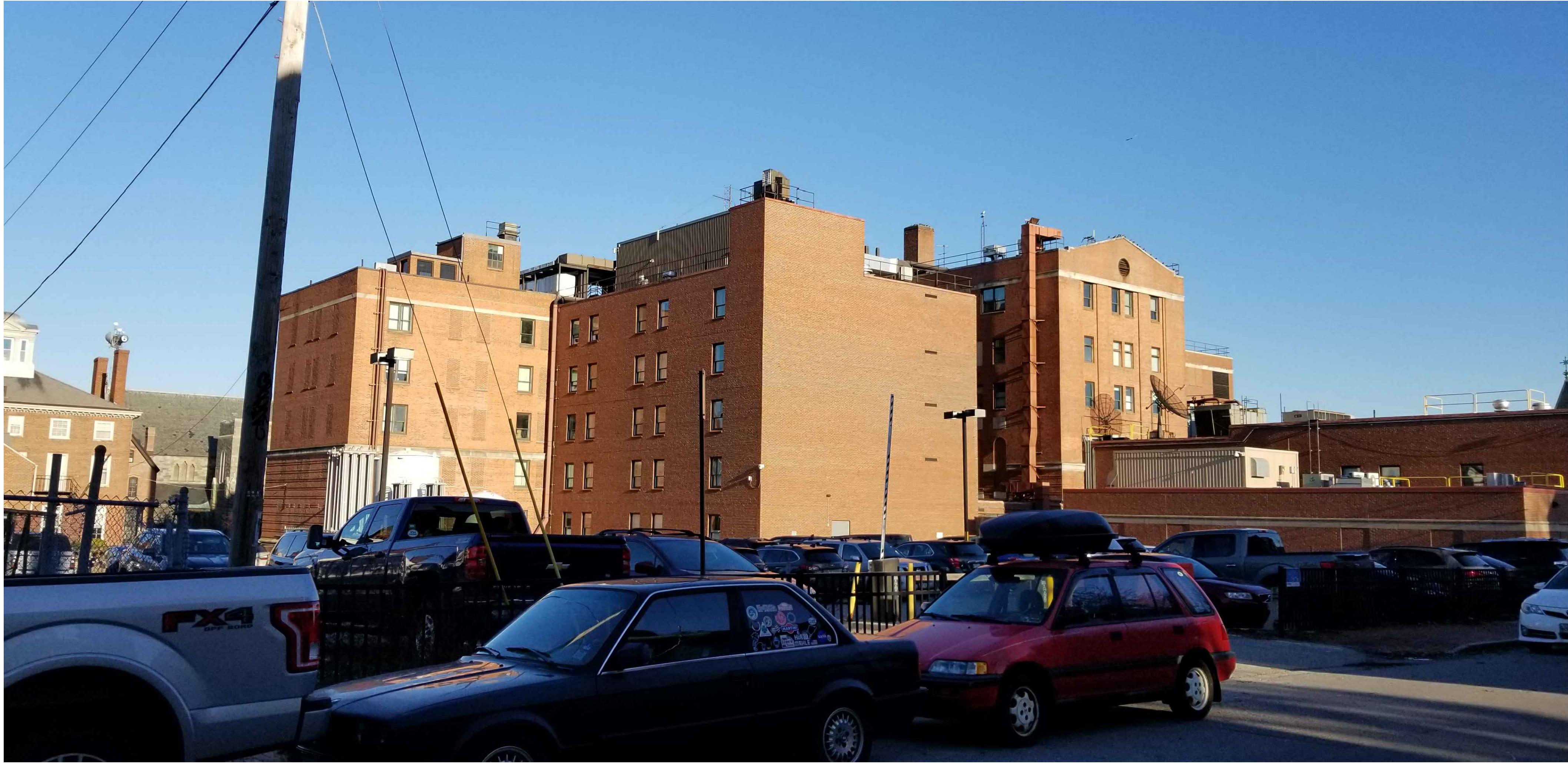
2 VIEW LOOKING EAST FROM WINTER ST.
