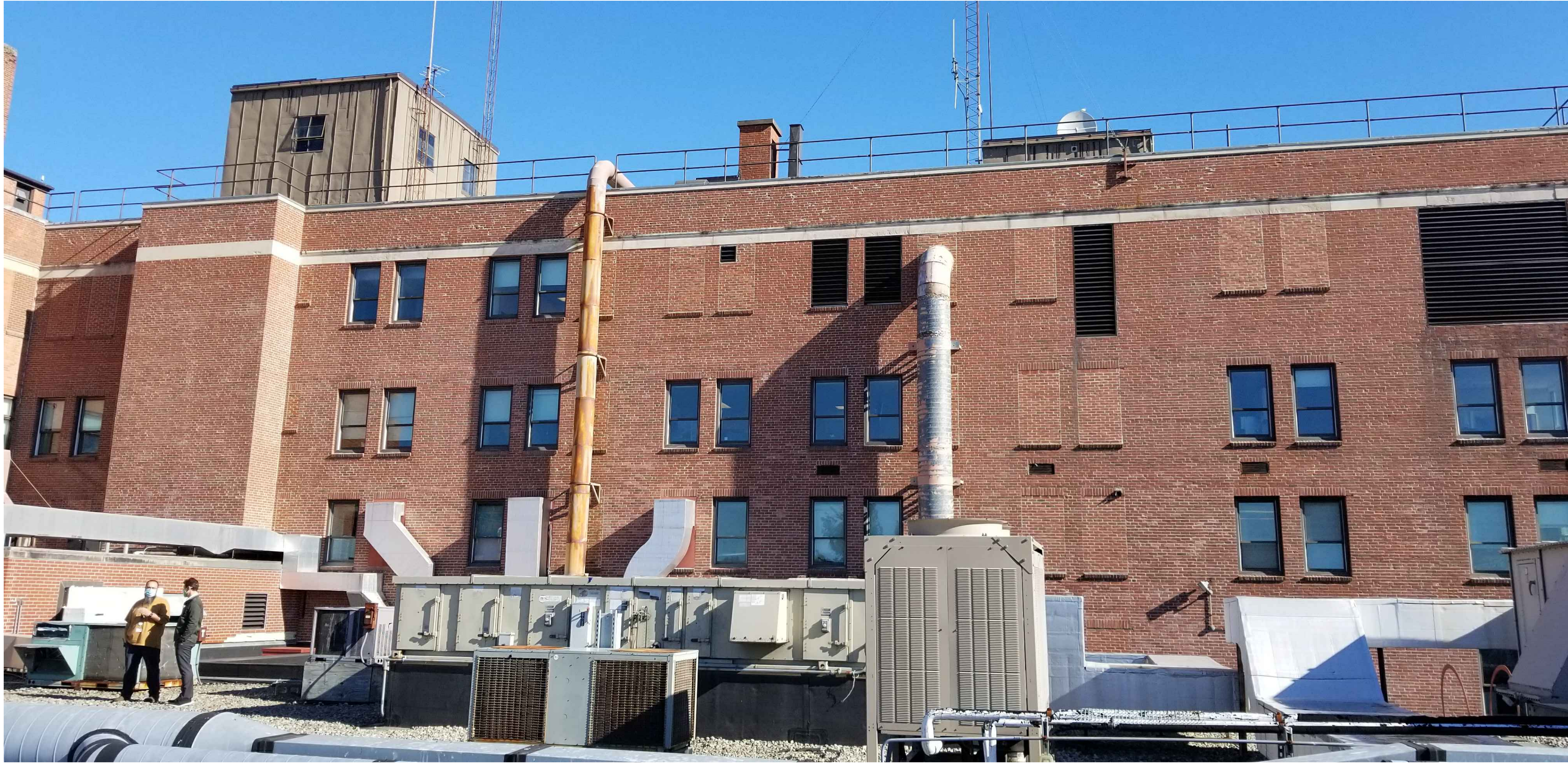
1 VIEW LOOKING NORTH / NORTH EAST FROM EMERGENCY ROOM ROOF KTS
