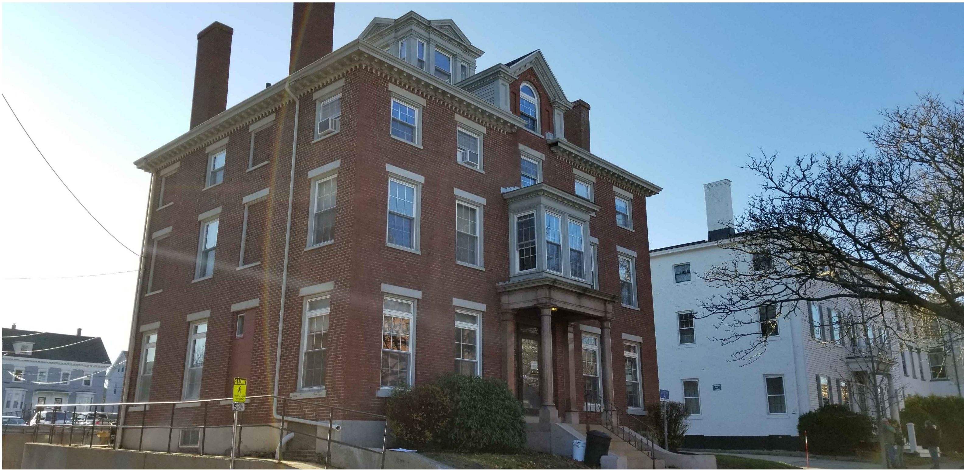
1 VIEW LOOKING SOUTH-WEST - EXISTING CONDITIONS
