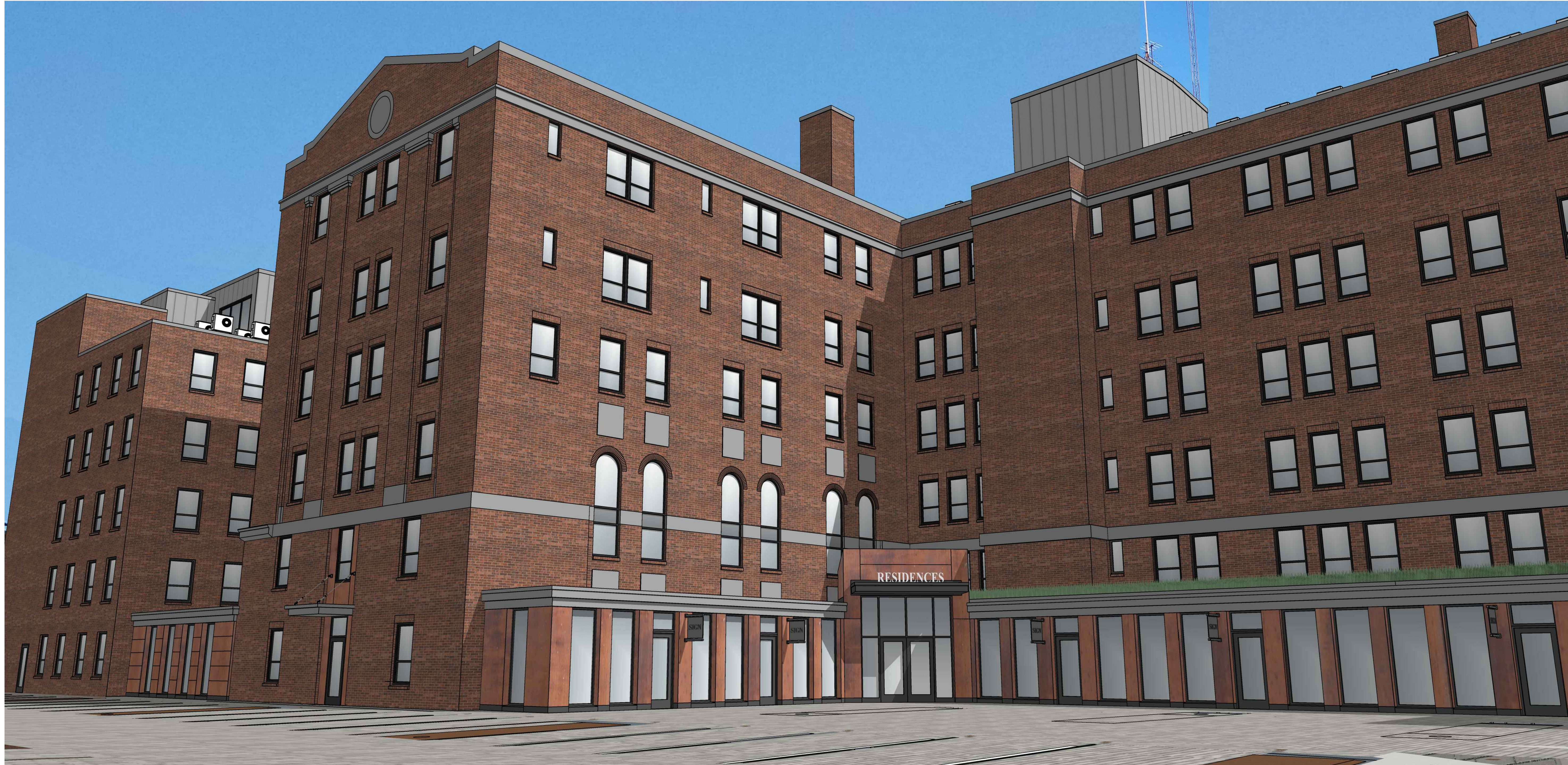
2 VIEW LOOKING NORTH FROM COURTYARD RTS
