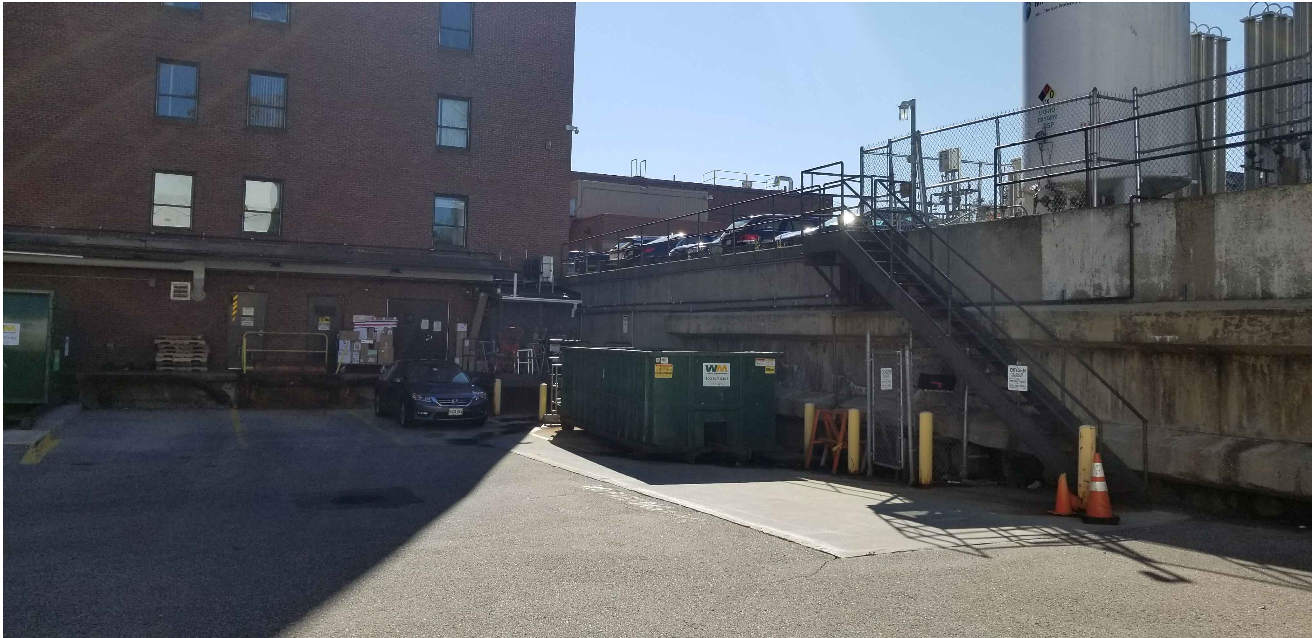
4 VIEW LOOKING EAST FROM LOADING DOCK AREA KTS
