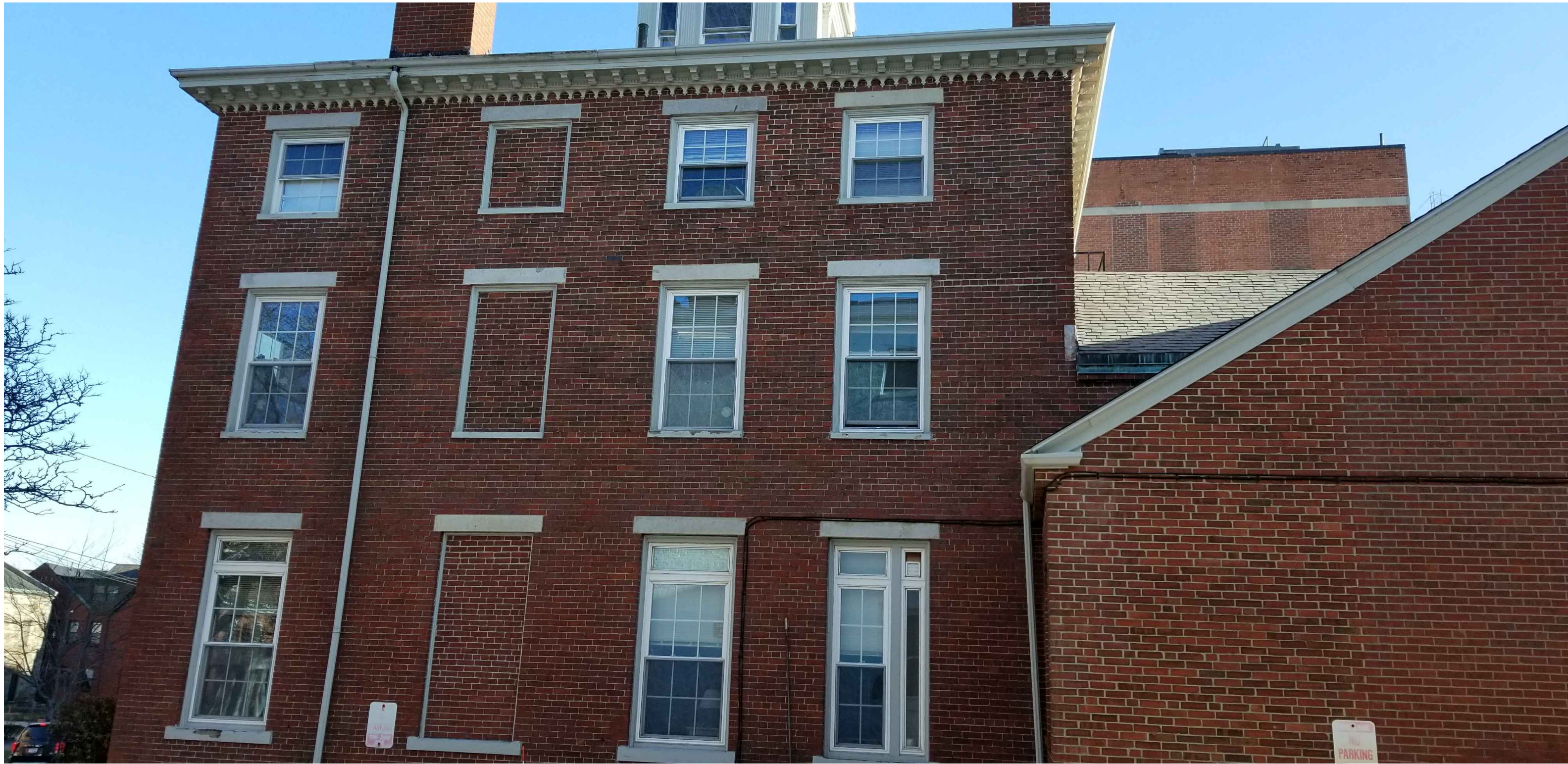
1 VIEW LOOKING EAST - EXISTING CONDITIONS
