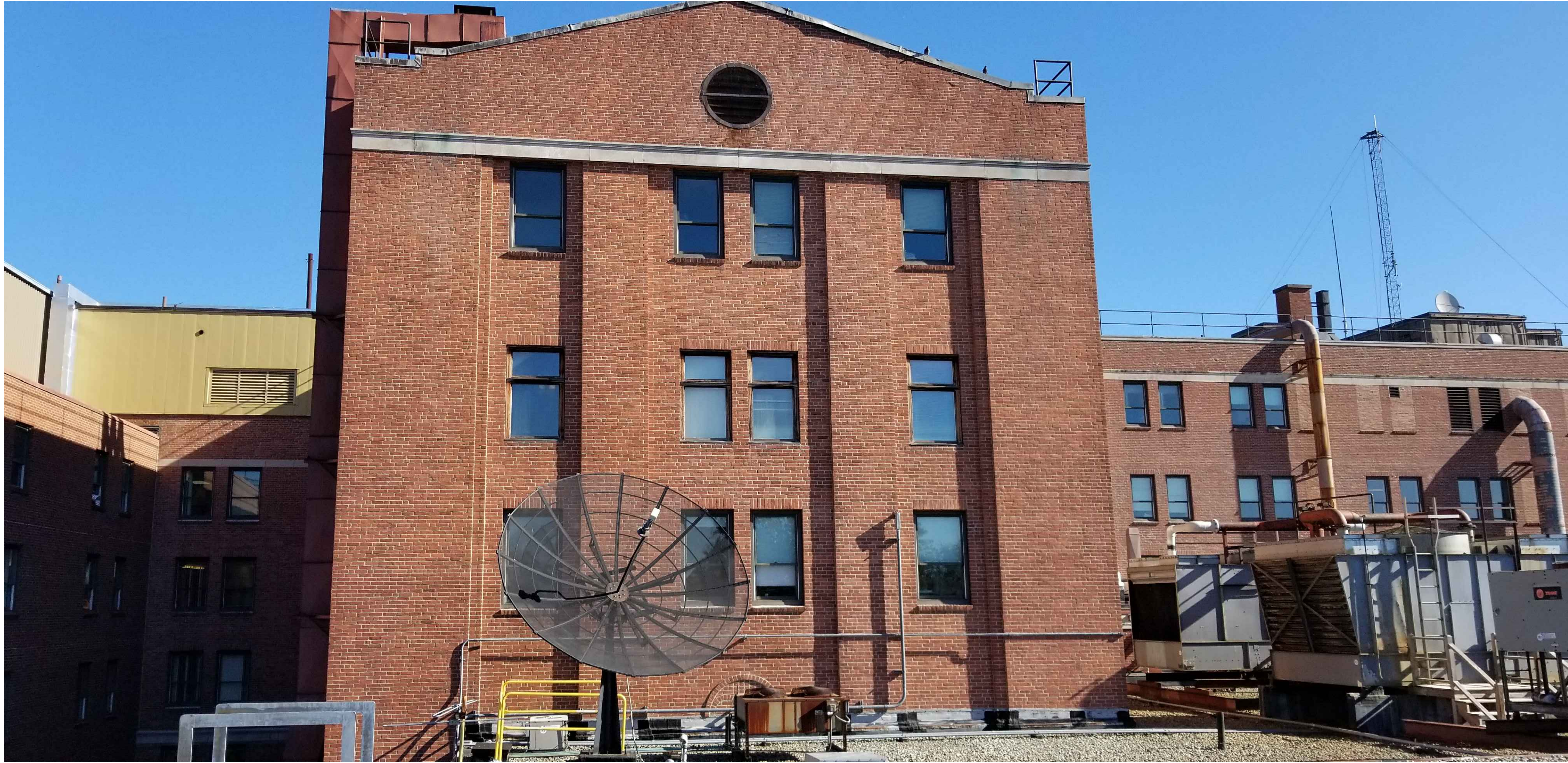
1 VIEW LOOKING NORTH-EAST FROM EMERGENCY ROOM ROOF KTS
