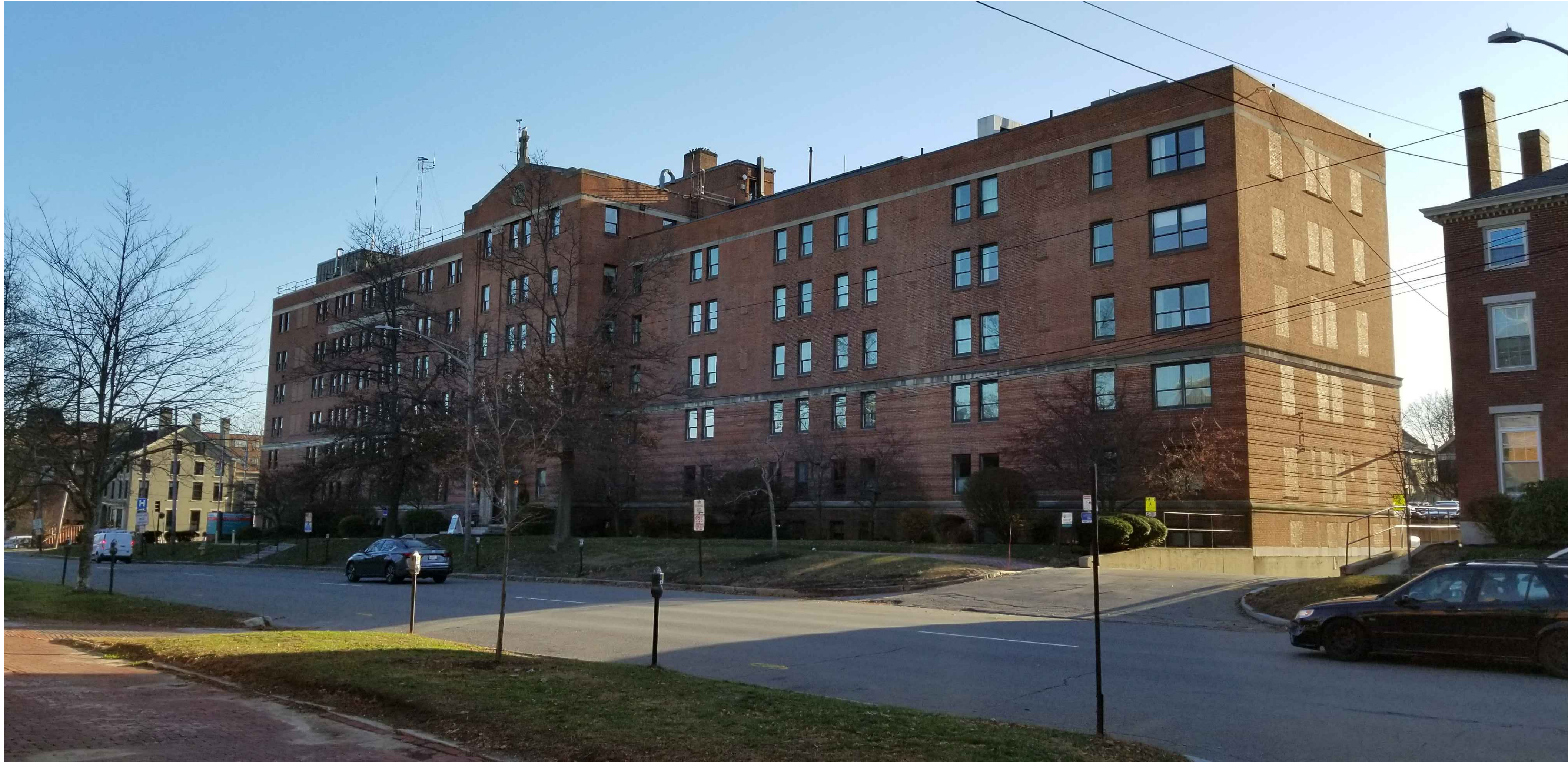
2 VIEW LOOKING SOUTH FROM STATE ST. KTS
