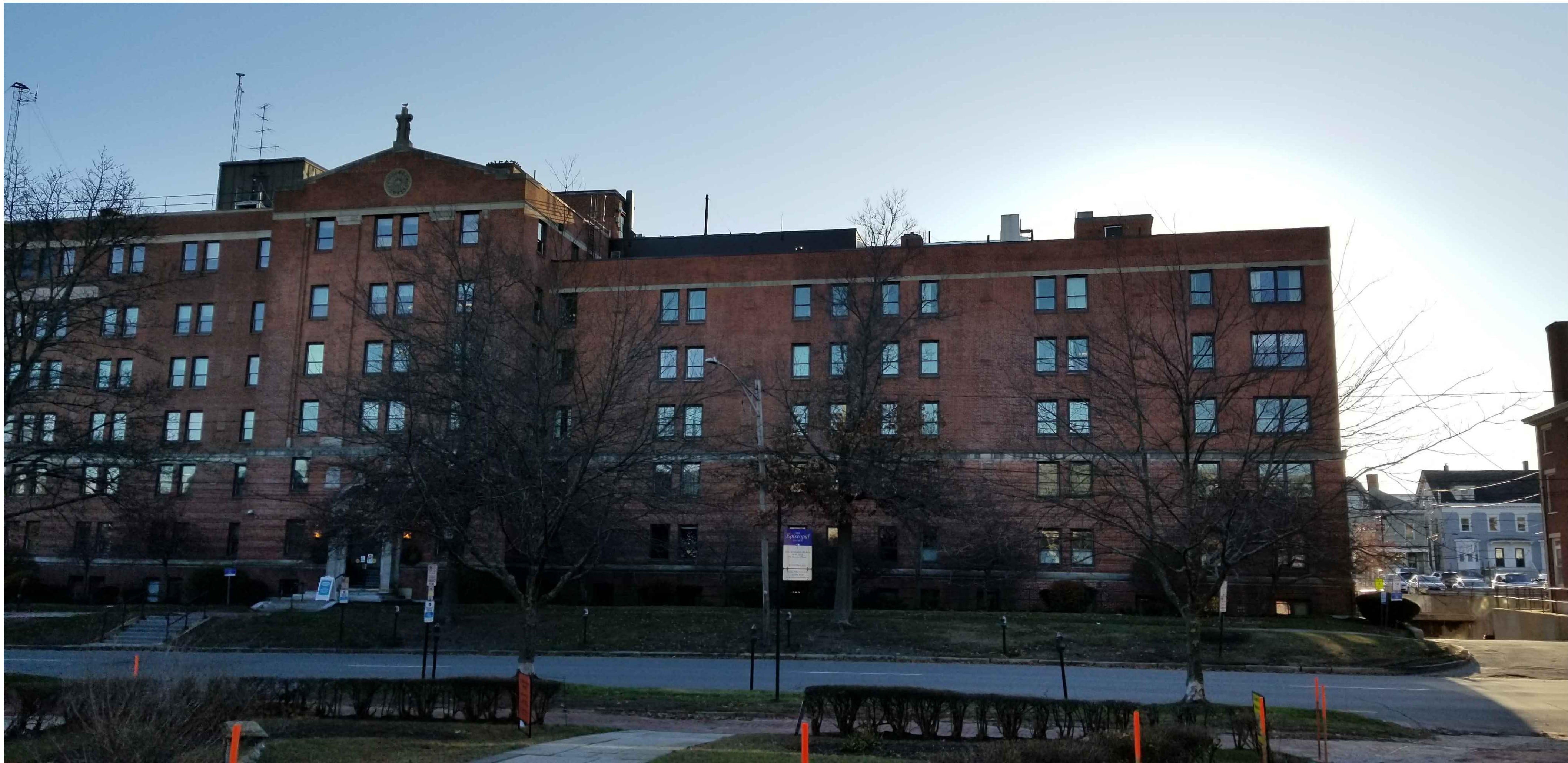
4 VIEW LOOKING SOUTH-WEST FROM ST. LUKE'S CATHEDRAL KTS
