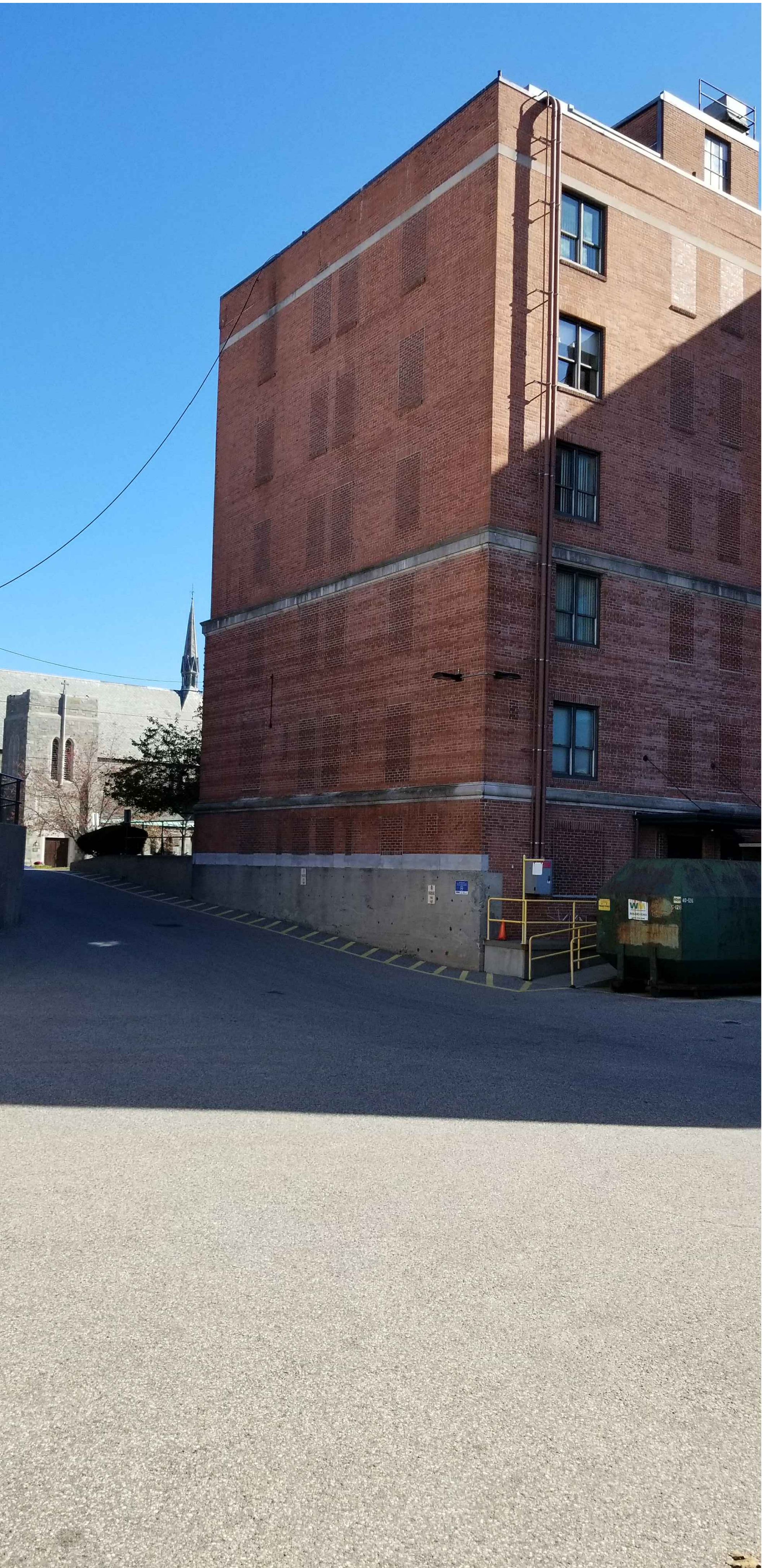
3 VIEW LOOKING NORTH-EAST FROM LOADING DOCK AREA N.T.S.
