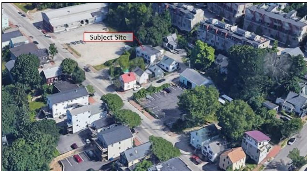
Figure 1 - Aerial view of 163 Washington Avenue
