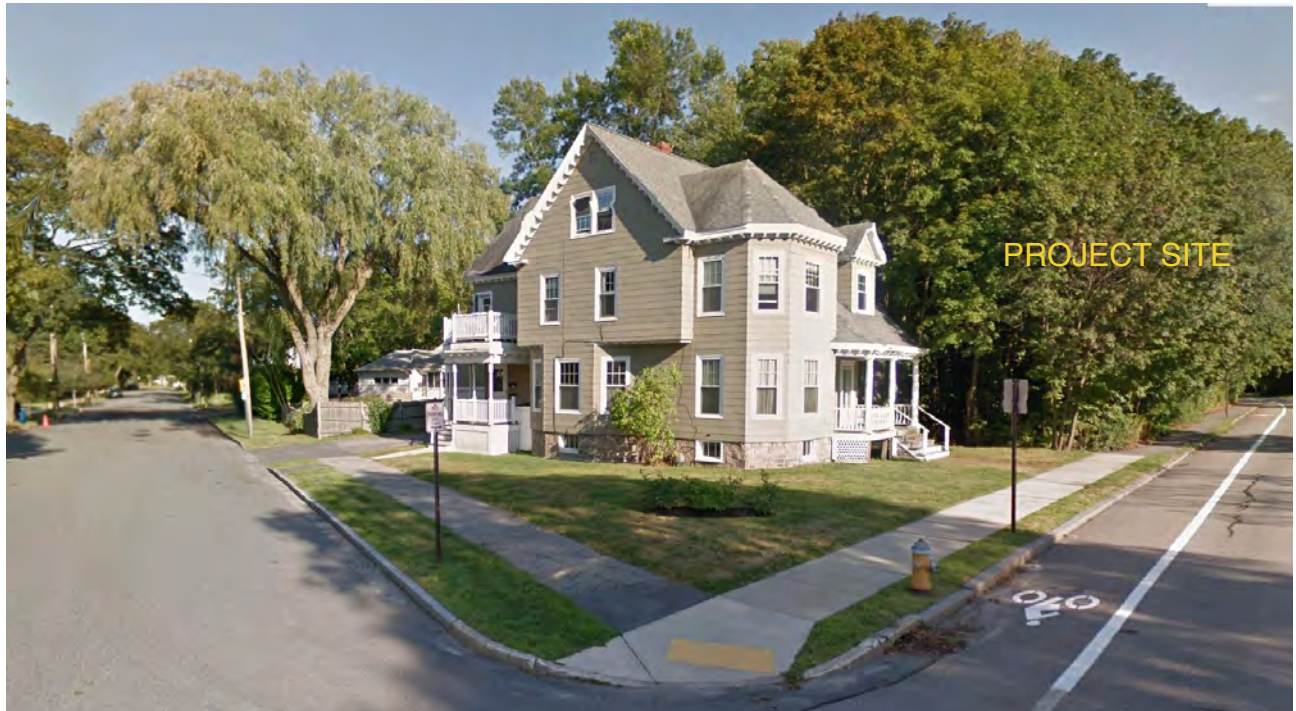
Two and a half story residence abutting the site at the corner of Deering Ave & Longfellow Street
