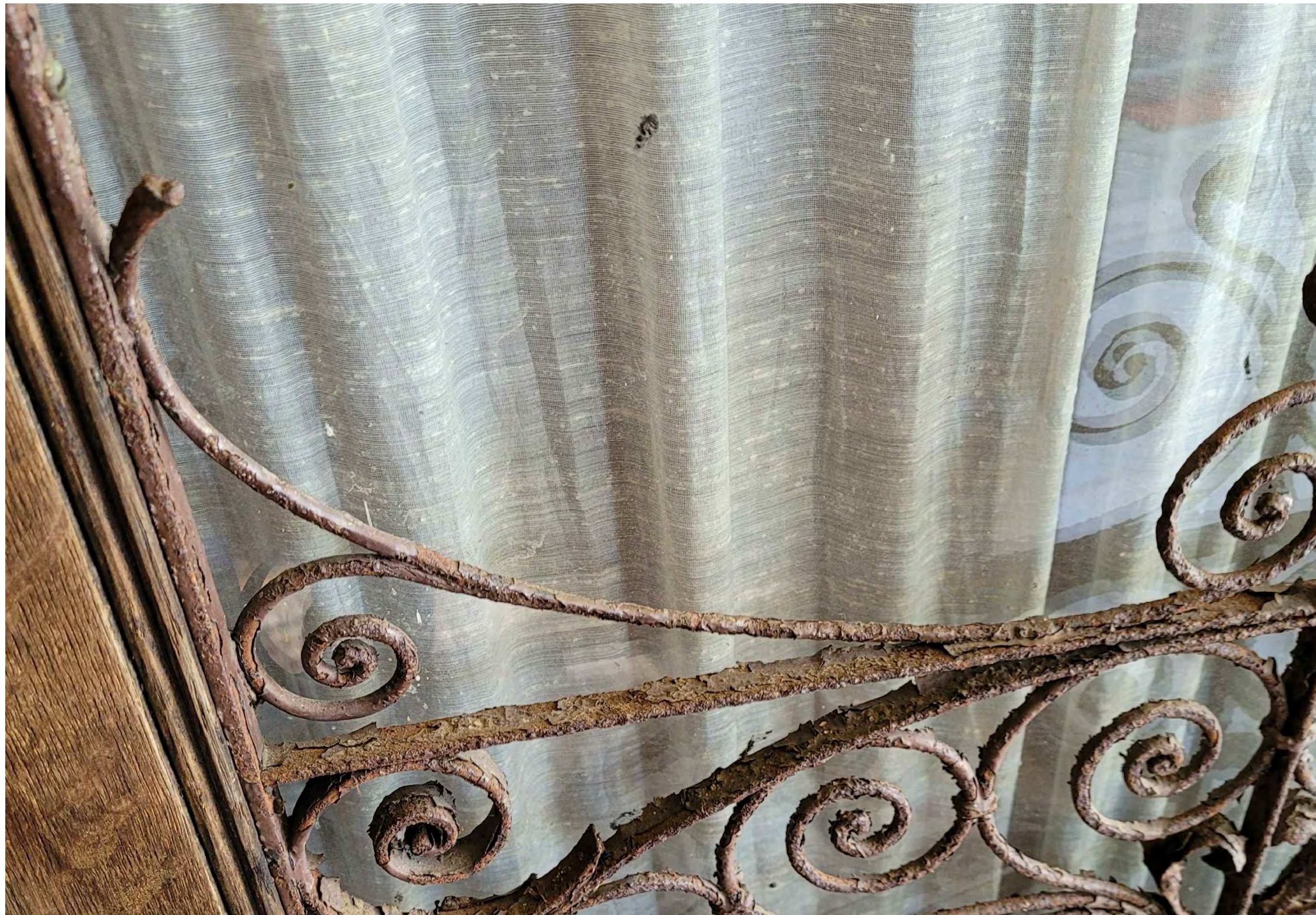
M. CORNER OF GRILLE TO BE REMOVED, FROM NORTH ELEVATION.
