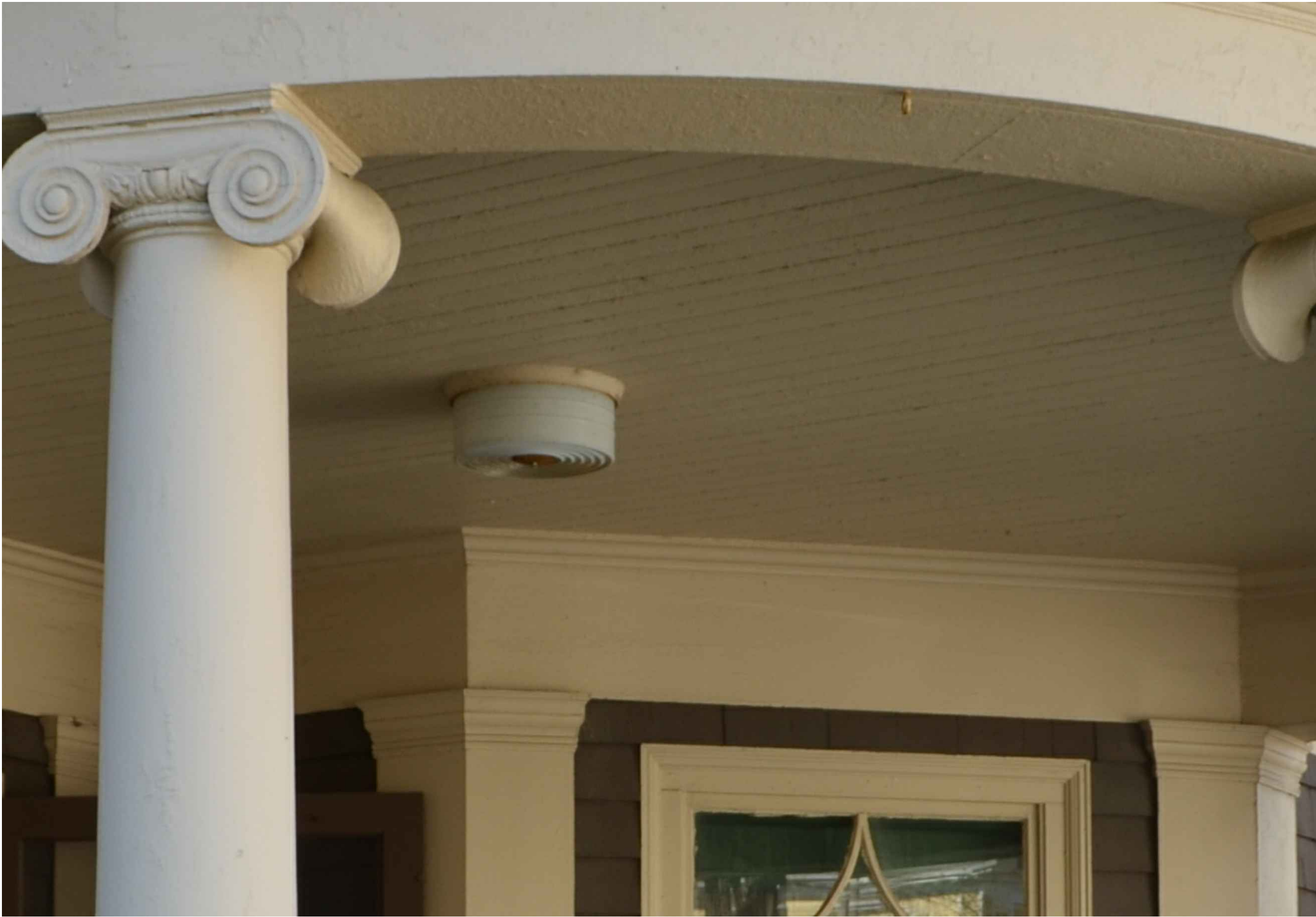
K. MODERN LIGHT FIXTURE ON PORCH TO BE REPLACED, FROM NORTH ELEVATION.
