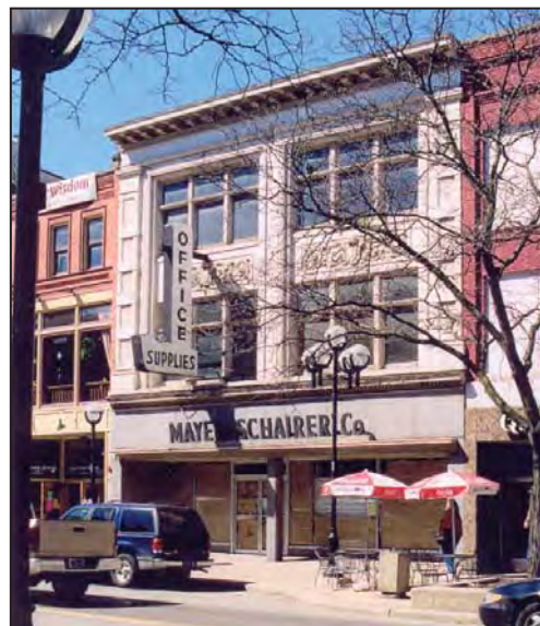
Three-story commercial building prior to rehabilitation.
