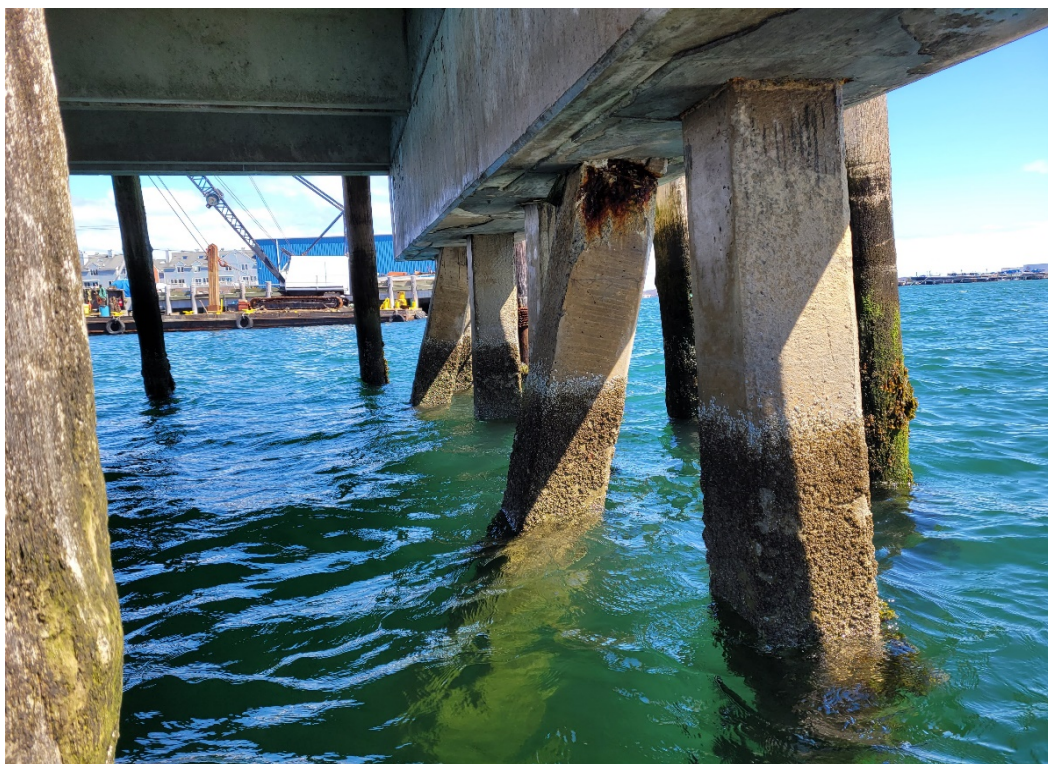
Picture #27 Sorting Pier 1 Extension, Bent 5
