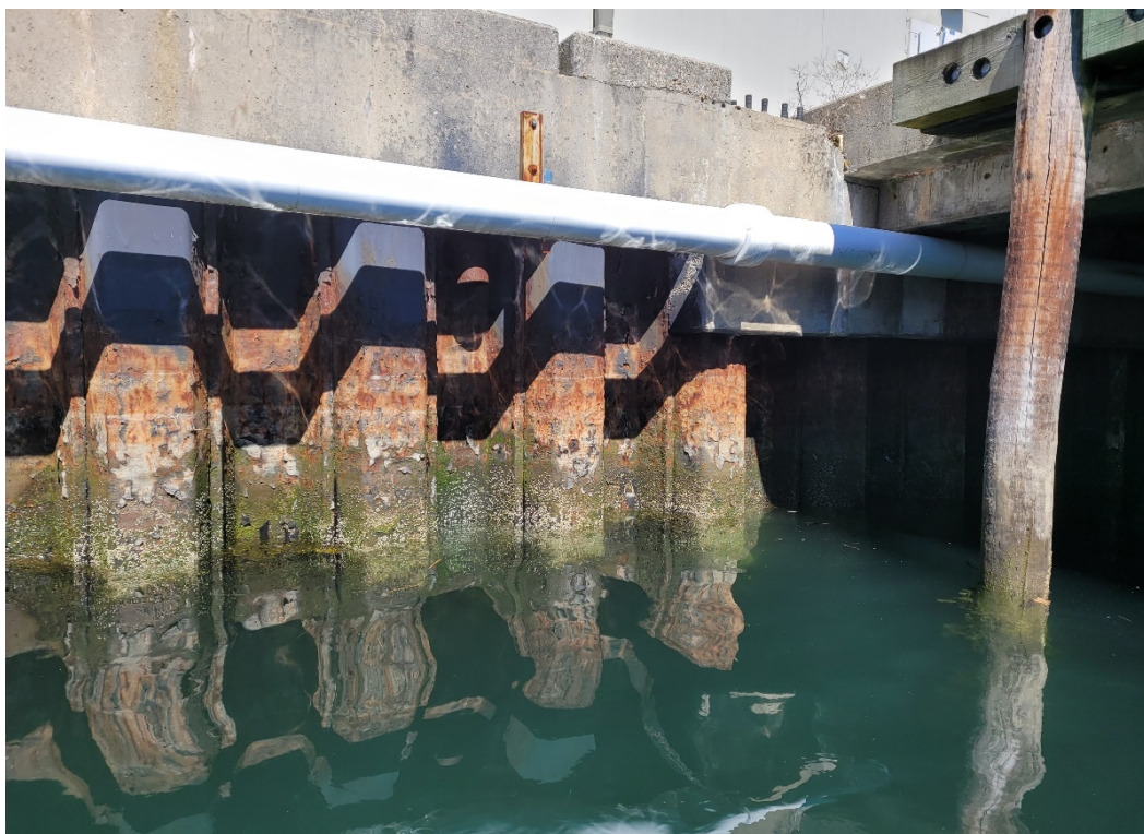
Picture #5 Typical sheet pile conditions between sorting piers
