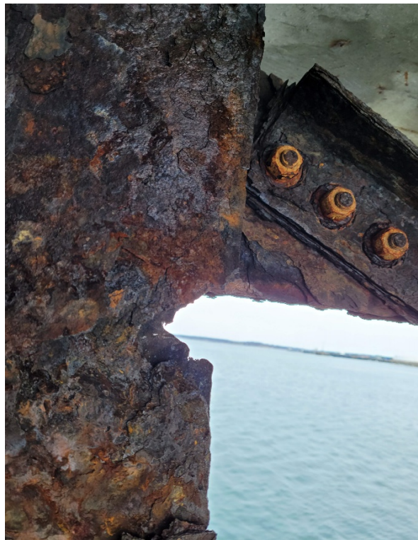
Picture #23 Service Pier 1, Bent 5, Pile 2
