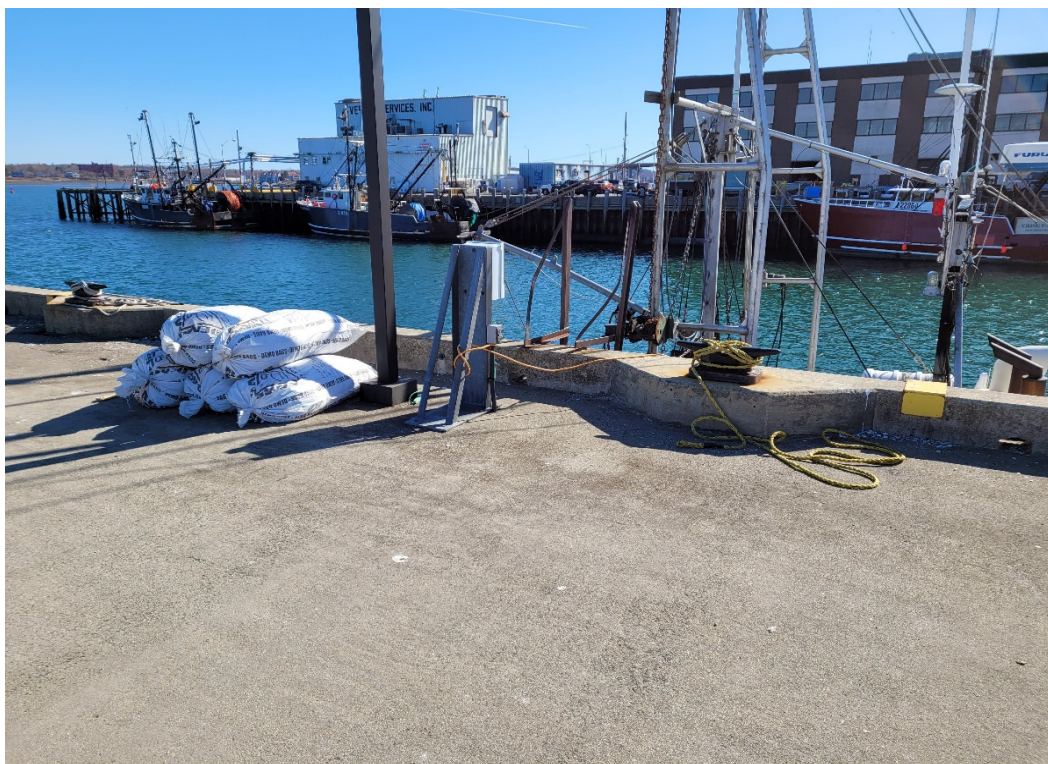
Picture #9 Deck of Sorting Pier 1 Extension
