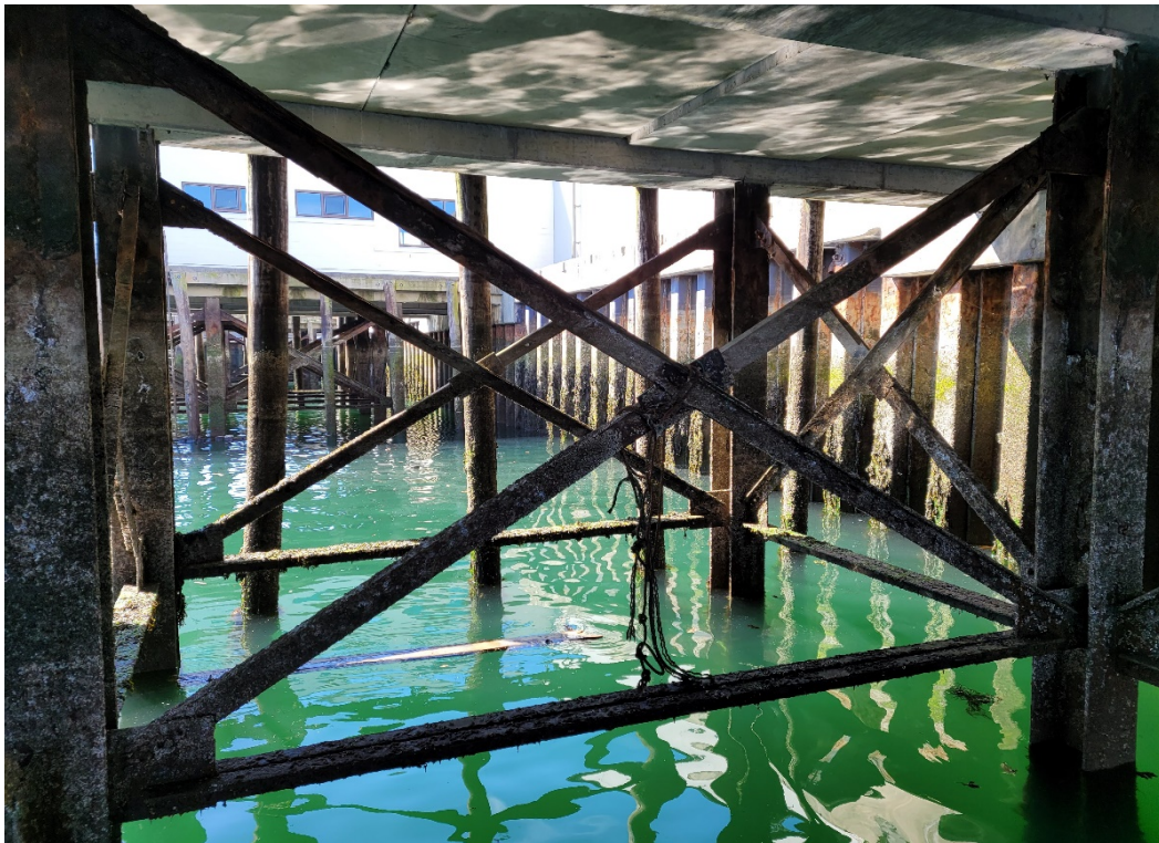
Picture #13 Typical bracing
