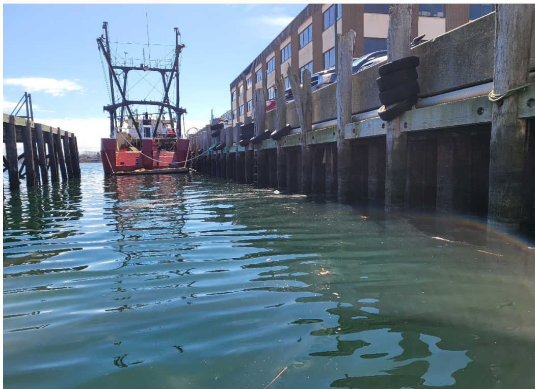
Picture #6 Looking south along east side of main pier
