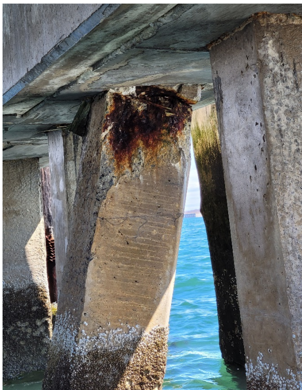
Picture #28 Sorting Pier 1 Extension, Bent 5, Pile 5
