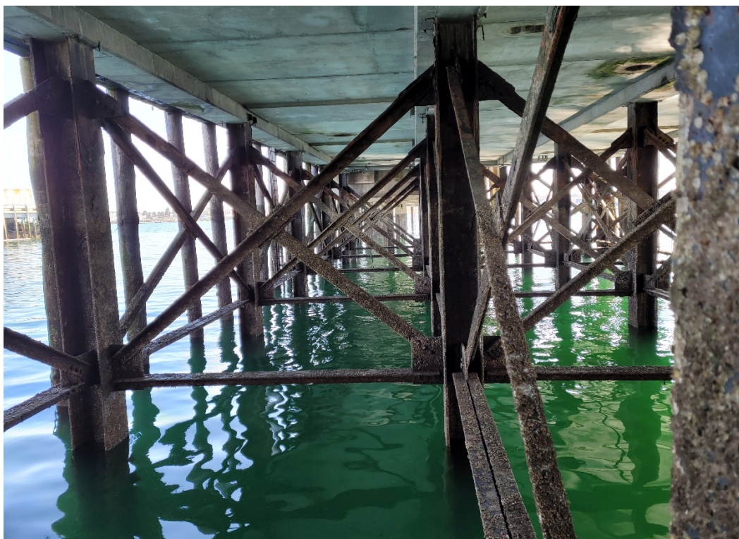
Picture #11 Looking south at Sorting Pier 1 Bent 2
