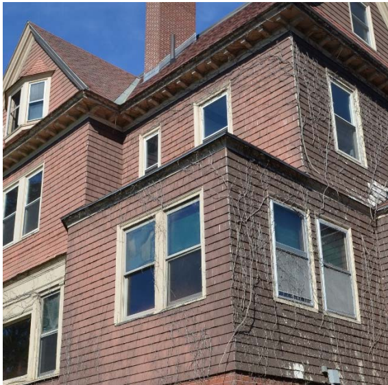
Existing Roof Area (New Deck)
