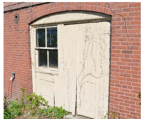
Arched Opening at Lower Level
