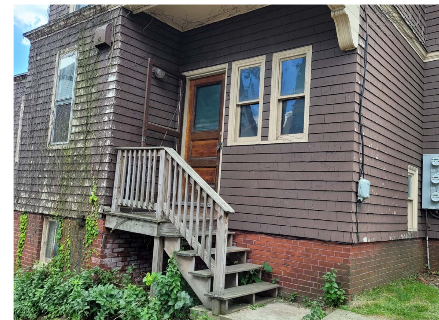
EXISTING LANDING AND STAIR TO BE REMOVED / REPLACED
