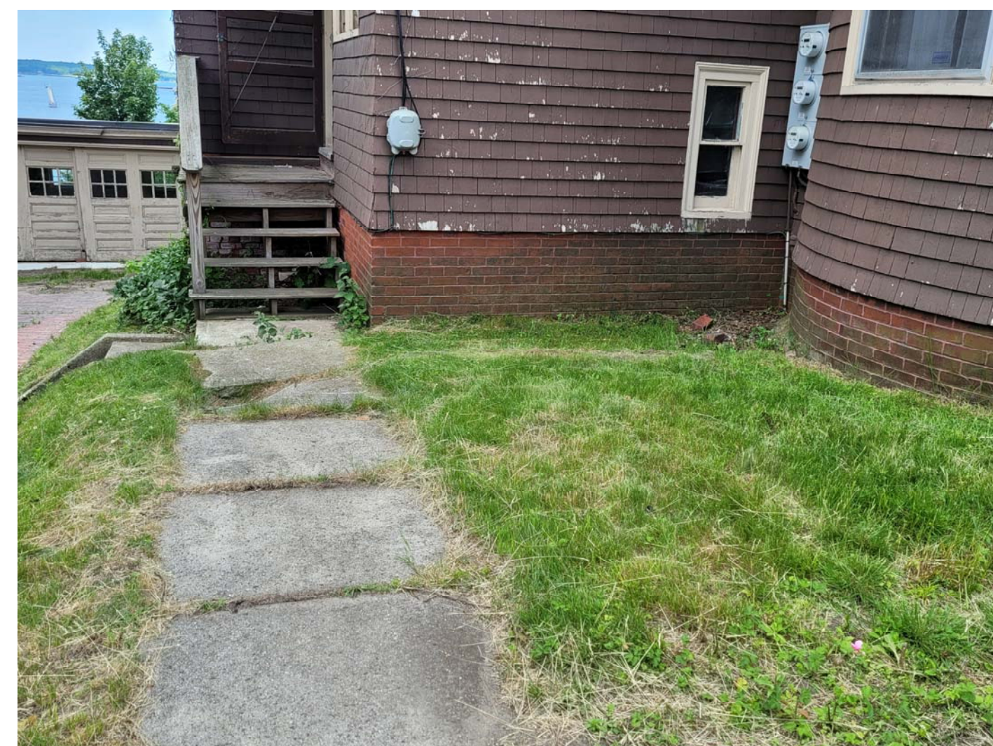
EXISTING SIDEWALK REPAIR
