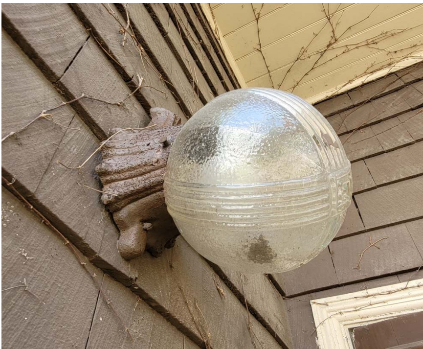
Fixture at side porch to be restored
