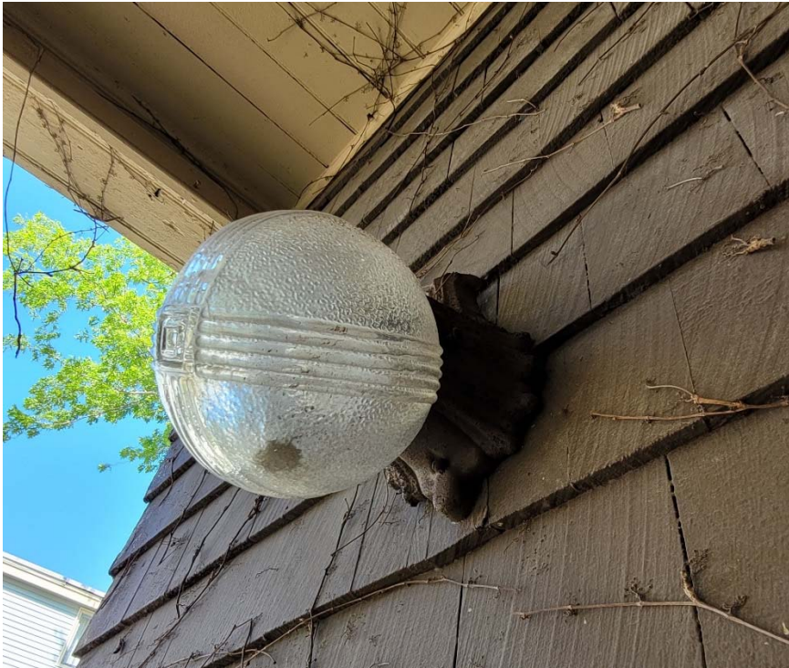
Fixture at side porch to be restored
