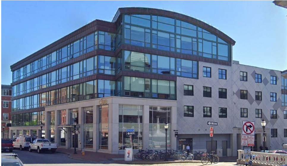
Figure 3: Existing Conditions (Image of Building Front) Source: Google Earth
