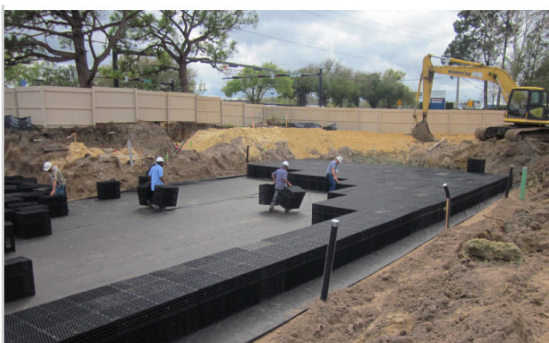
Fig 3. R Tank Underground Storage
