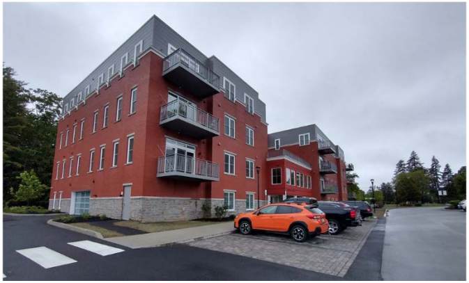
Figure 4: Stevens Square Building 1
