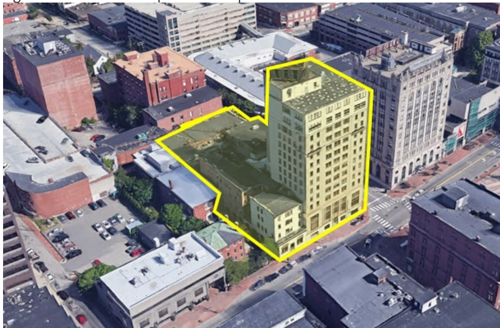
Figure 1 - Aerial of the Proposed Development
