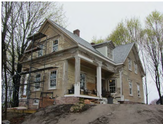
99 Capisic Street, during 2021 rehabilitation
