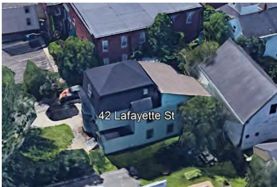
Aerial view, looking southwest. Note addition off north elevation.
