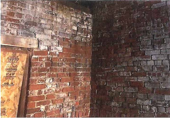
Separating Building #12 Wall from Common wall between 12 and 11
