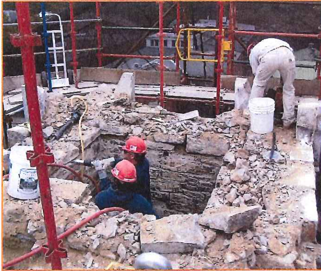
Disassembly of Veneer and Backup Wall
