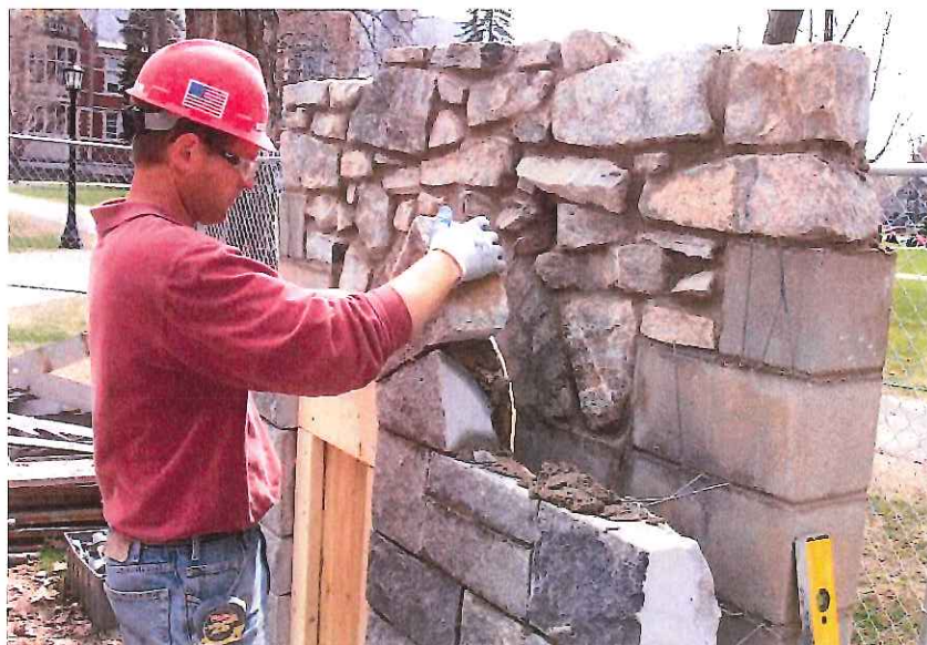
Preconstruction Mockups for Quality Control of coursing
