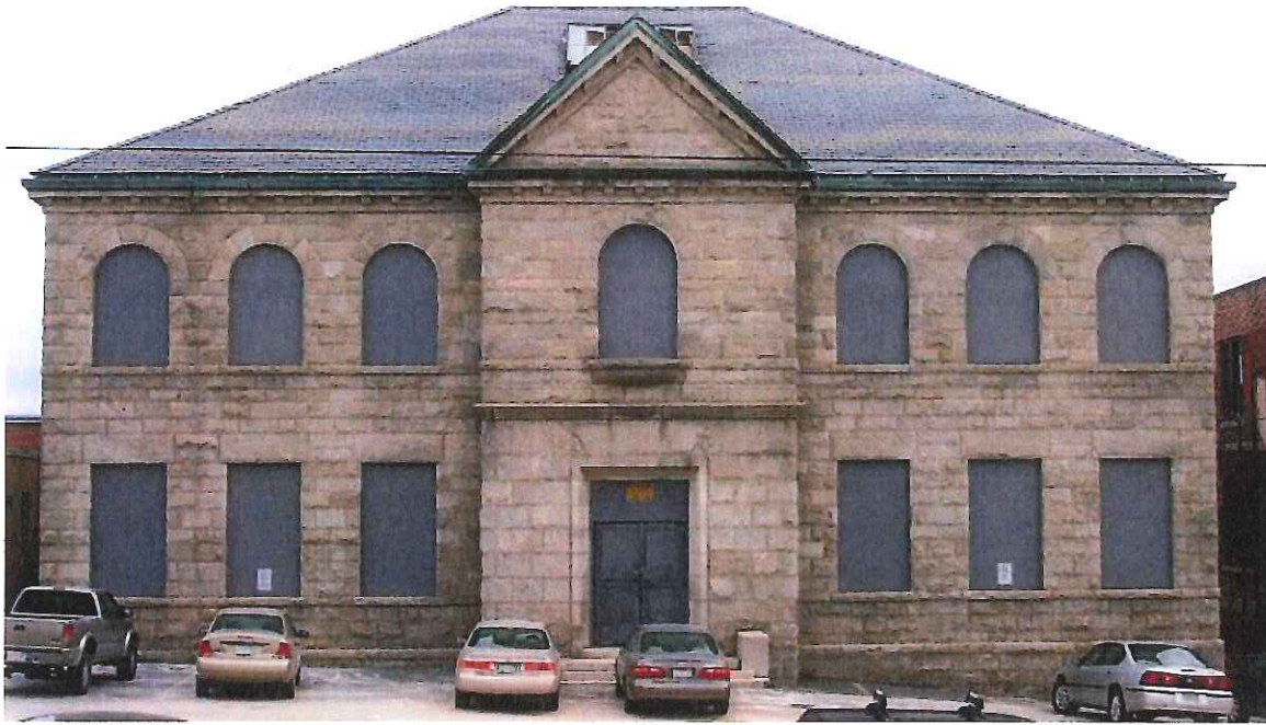
Granite Building Prior to Relocation – Suffered significant Fire in 1985 and Boarded Up
