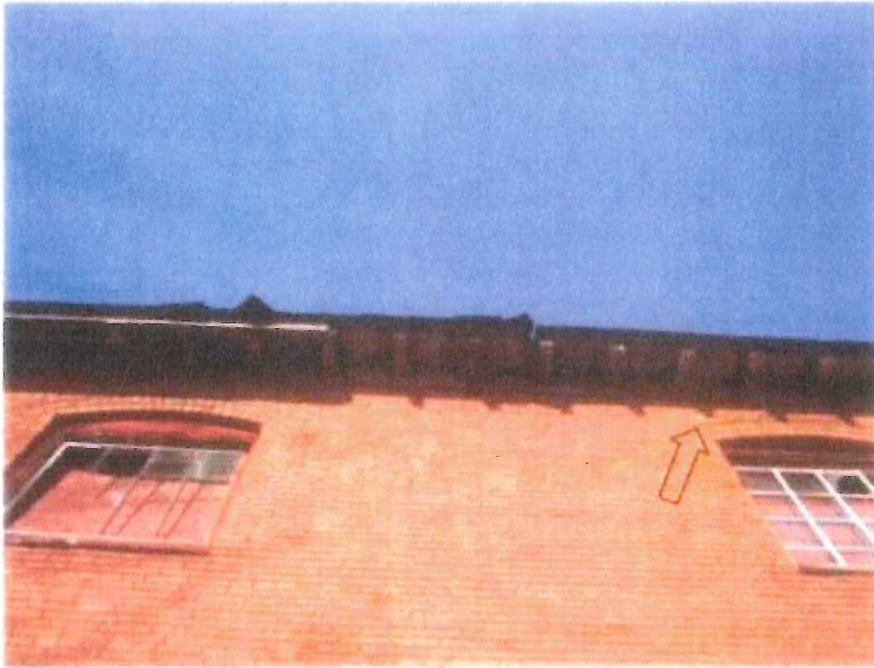
Photo 12-2: Eave with loose slates, missing eave trim, masonry cracking and broken windows.
