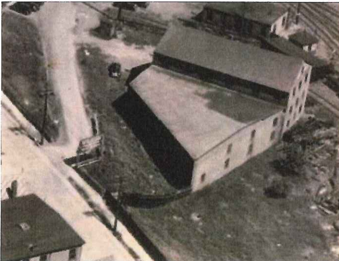
Building #12 – South Elevation - Excerpted from source image above
