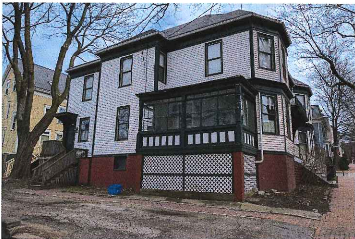
PHOTO OF THE EXISTING BUILDING
