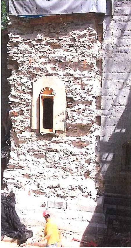
Disassembly of Lower Tower – Veneer Only
