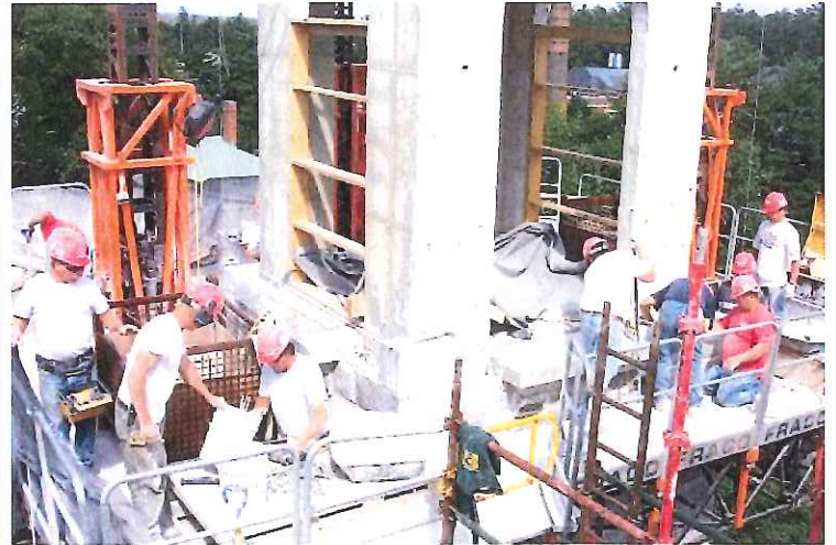
Reconstruction of Backup Wall – using Precast
