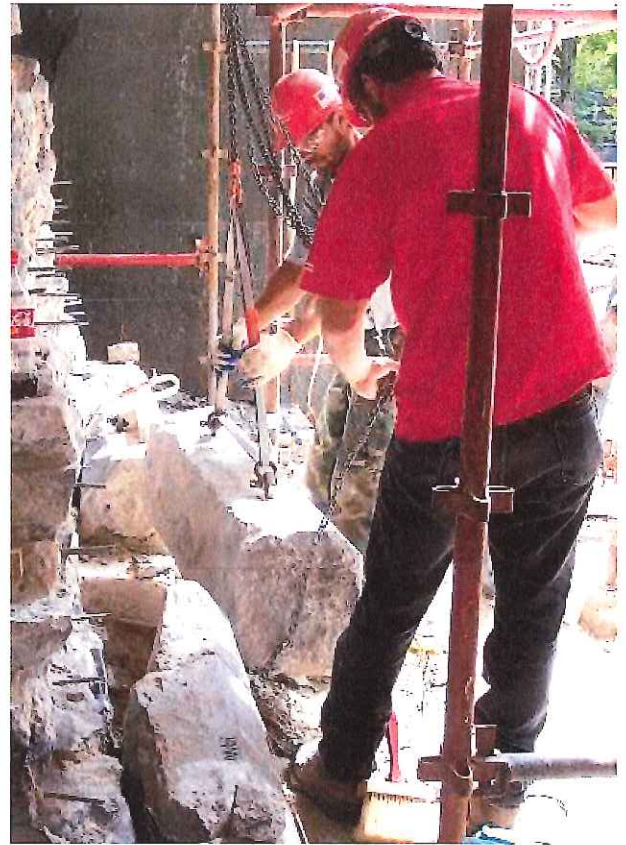
Reconstructed Veneer at Lower Towers
