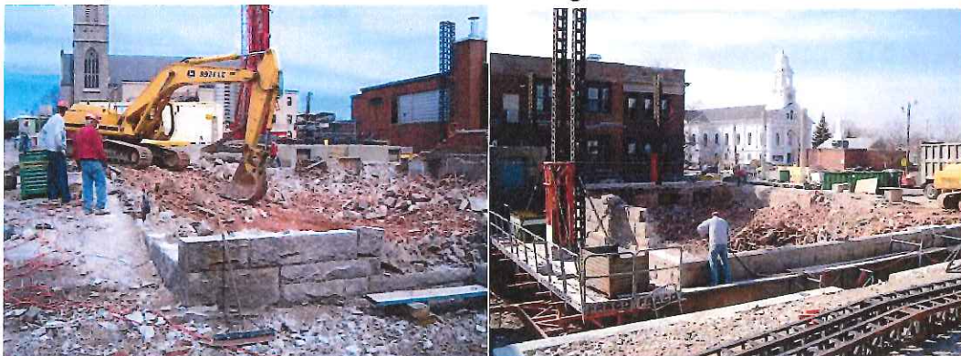
Salvaging Stone Veneer – Demolishing Backup wall Masonry
