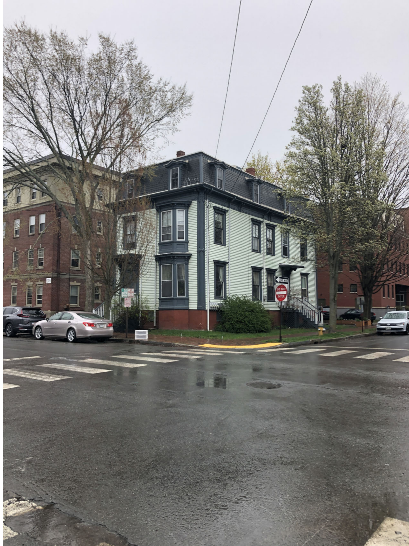
OVERALL STRUCTURE, NO VIEW OF PROPOSED DECK
