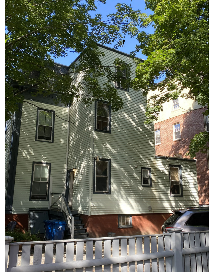
EXISTING REAR VIEW FROM CARLTON STREET
