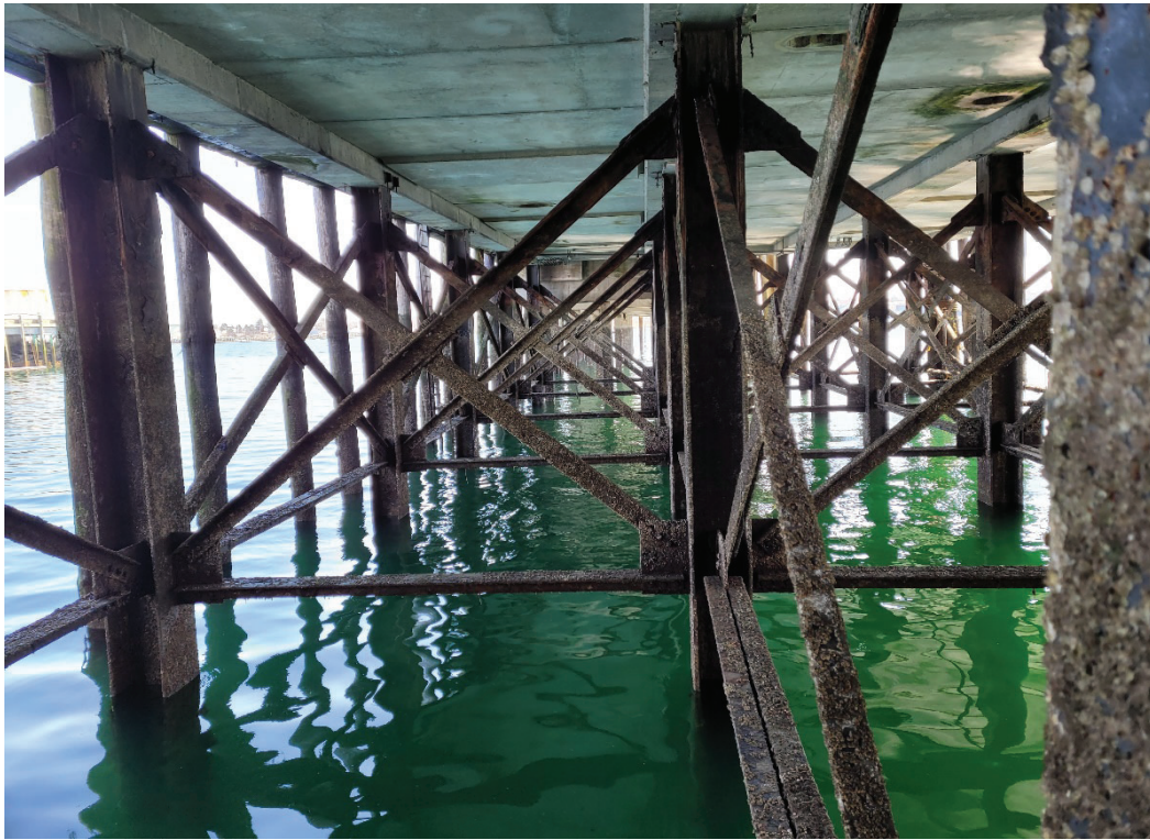
Picture #11 Looking south at Sorting Pier 1 Bent 2
