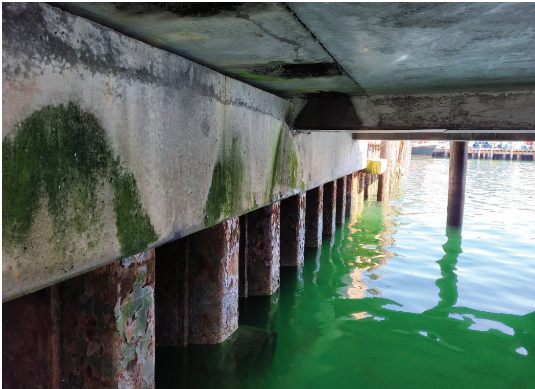
Picture #8 Typical sheet pile conditions beneath sorting piers
