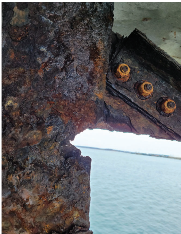
Picture #23 Service Pier 1, Bent 5, Pile 2
