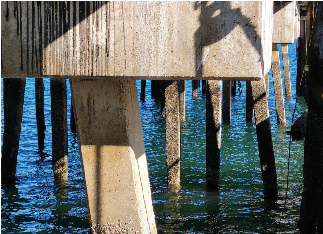
Picture #26 Sorting Pier 1 Extension
