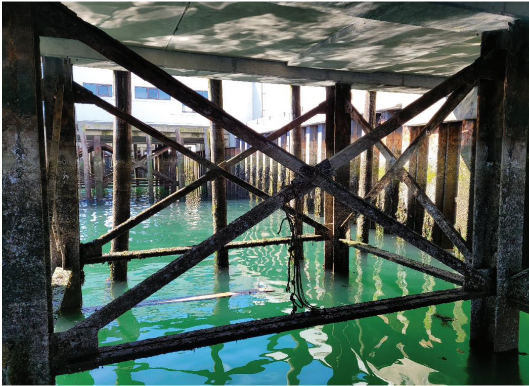
Picture #13 Typical bracing
