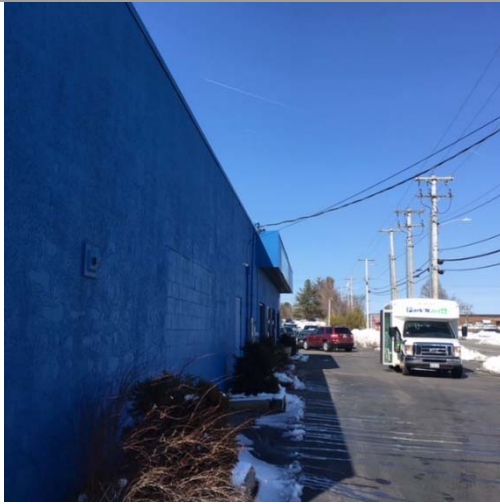
FRONT EXTERIOR VIEW
