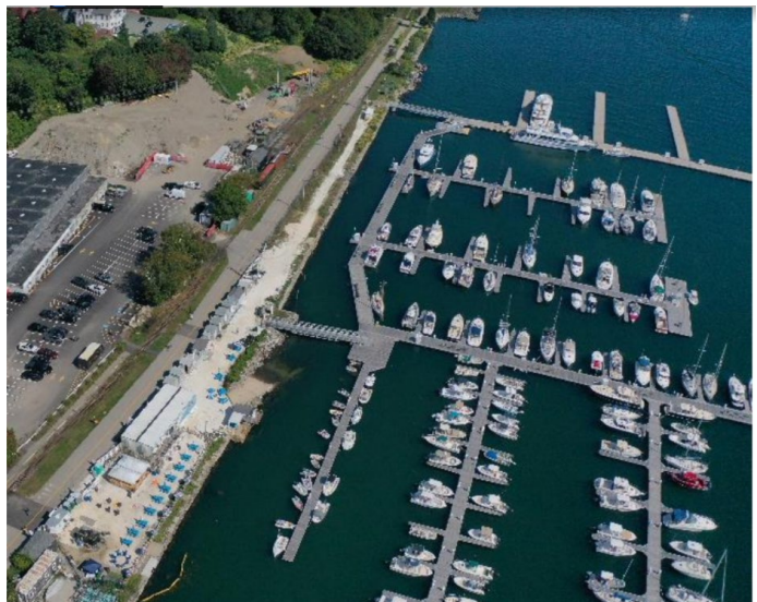
Figure 1: Aerial view of the Fore Points Marina and waterfront portion of the Portland Foreside Development
