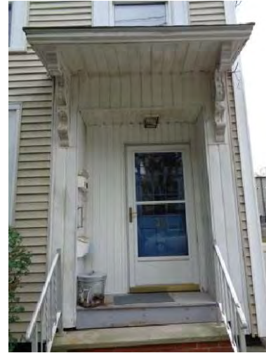
existing front entry
