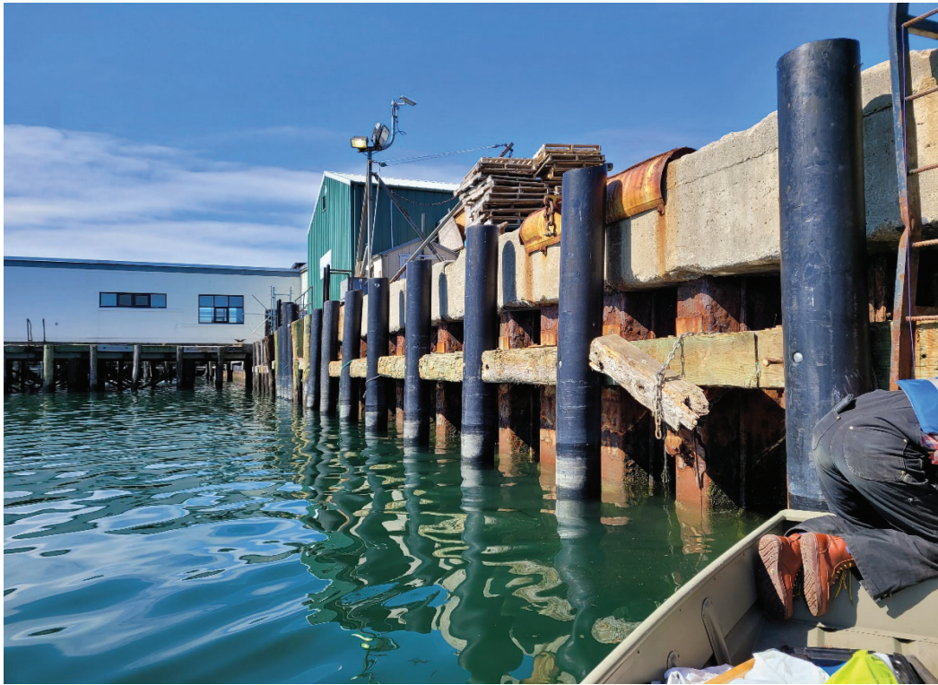
Picture #3 Looking West along south face of the Net Yard
