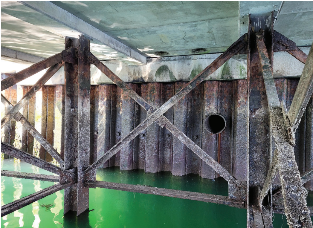
Picture #12 Looking north at Sorting Pier 1 Bent 1 and sheet pile
