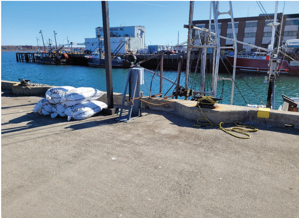
Picture #9 Deck of Sorting Pier 1 Extension
