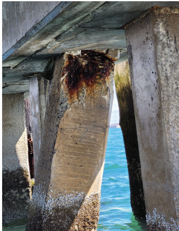
Picture #28 Sorting Pier 1 Extension, Bent 5, Pile 5
