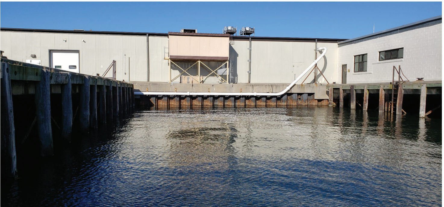
Picture #2 Looking north at the Fish Exchange between Sorting Piers 2 & 3
