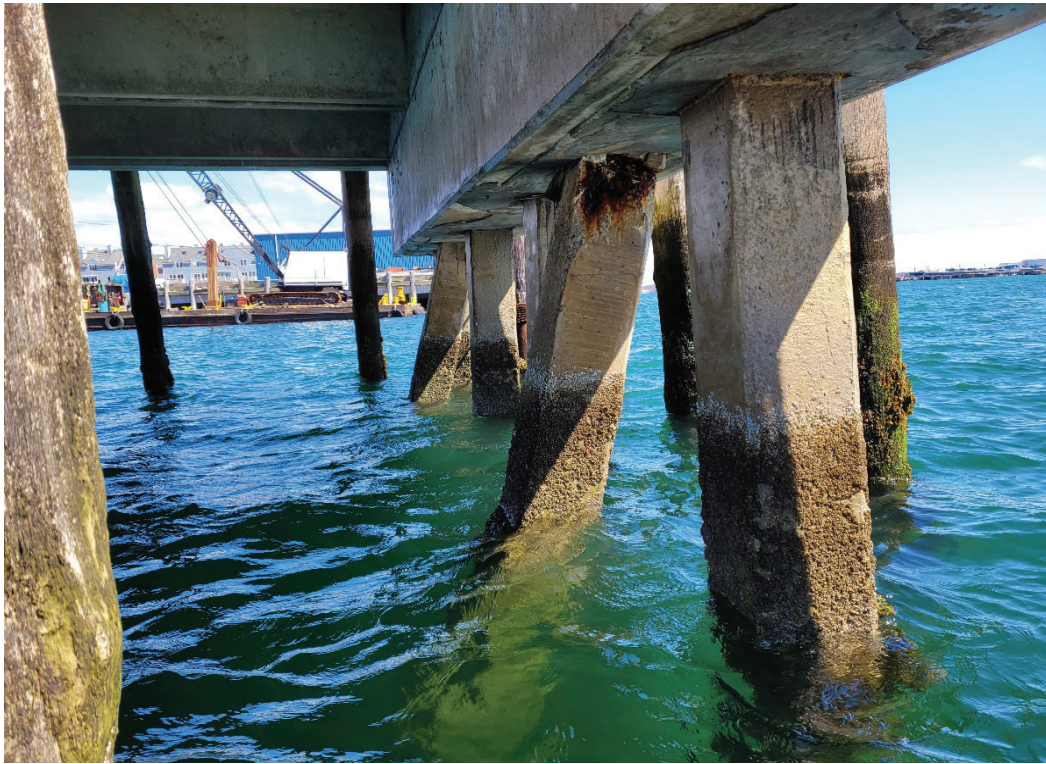
Picture #27 Sorting Pier 1 Extension, Bent 5
