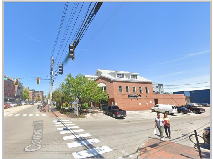
Figure 5: Google Street View of Union Wharf/Commercial
