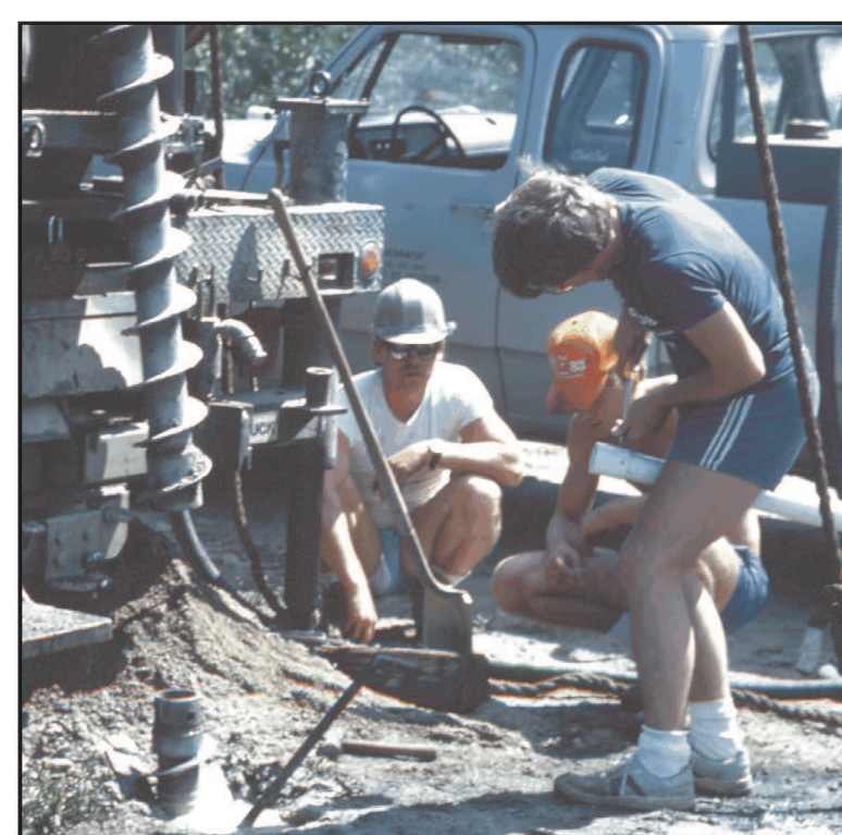
Installing a monitoring well, Washington County, Maine.
