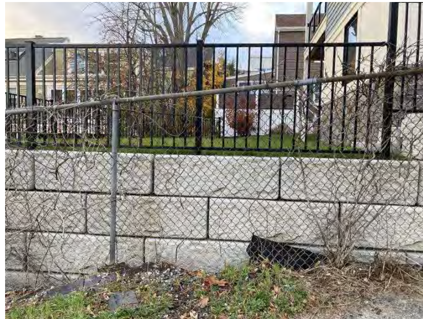
existing retaining wall & fence
