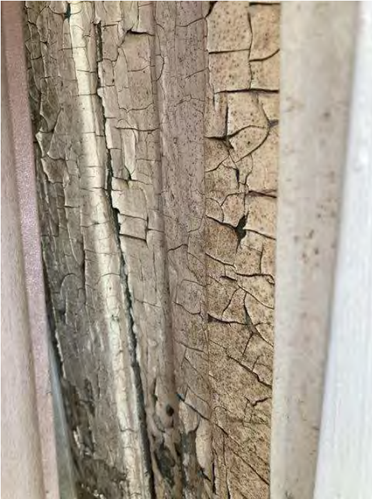
existing trim alongside door at front entry
