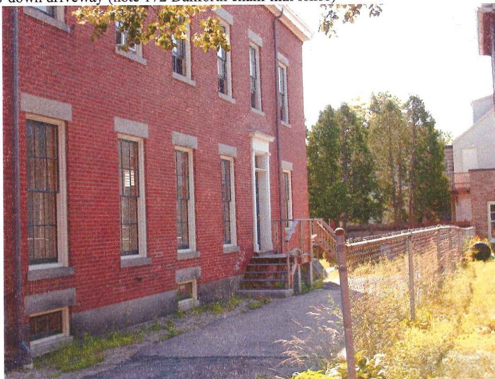
View down driveway (note 172 Danforth chain-link fence)
