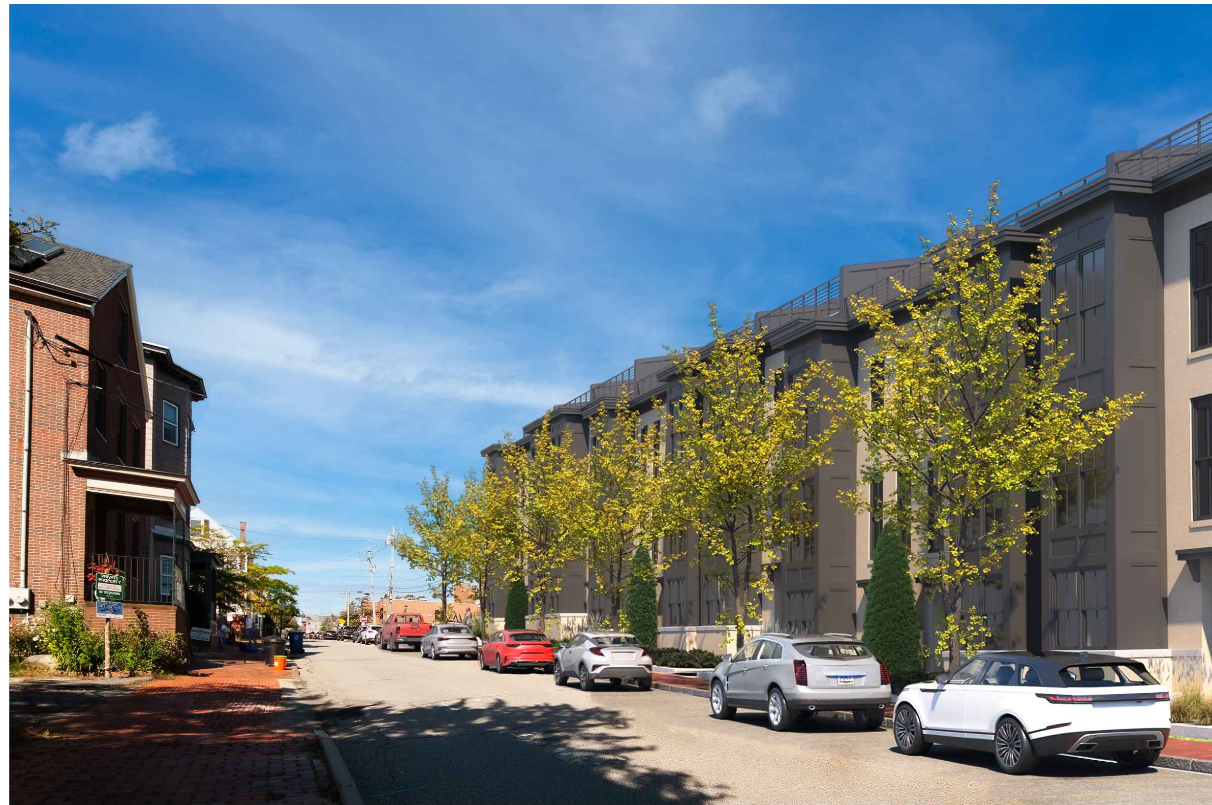
3 VIEW FROM DOWN WINTER STREET
