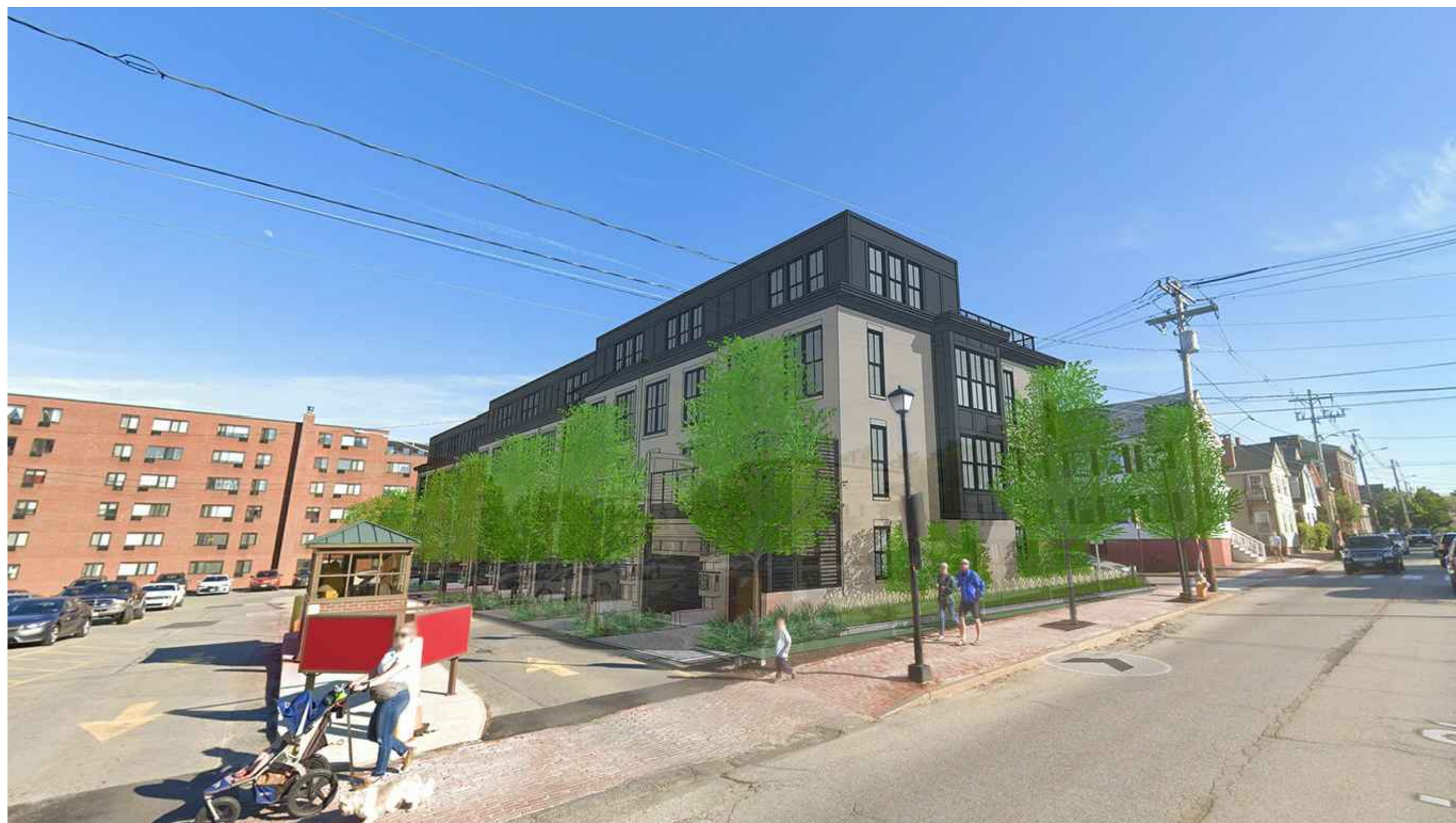
3 VIEW DOWN SPRING STREET
