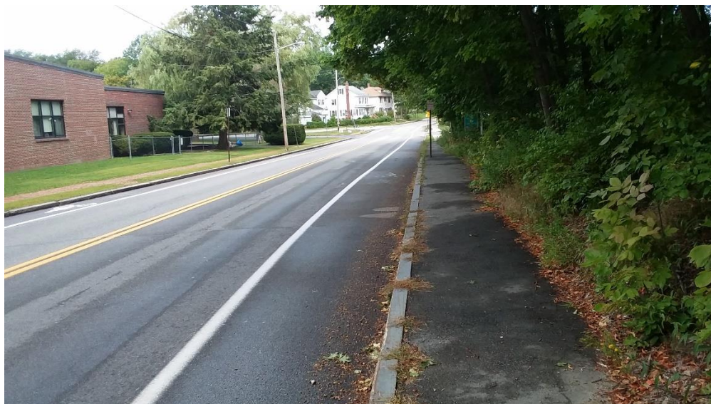
Representative image of existing sidewalk (9/11/2019)
