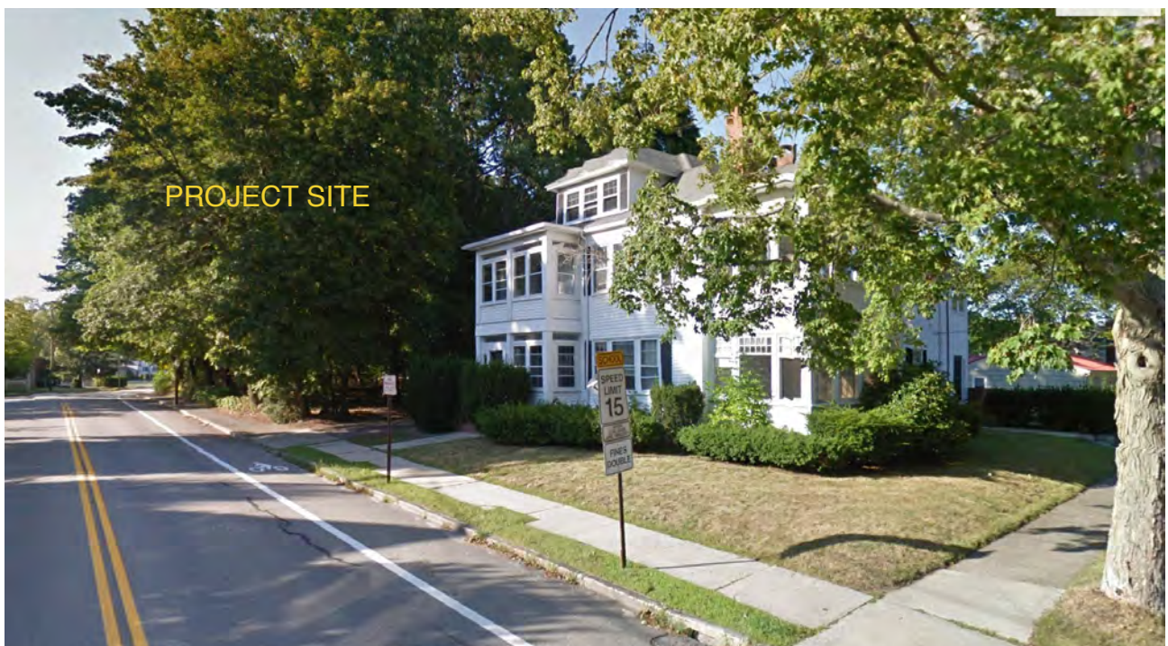
Two and a half story residence abutting the site at the corner of Deering Ave & Noyes Street
