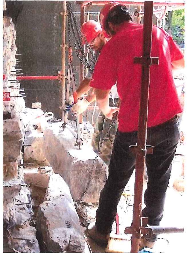
Reconstructed Veneer at Lower Towers
