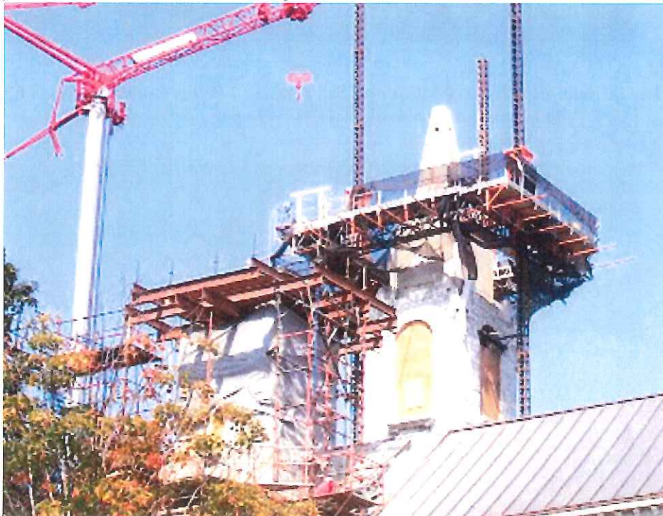
Reconstruction of Structural Backup at upper Belfry and Spires
