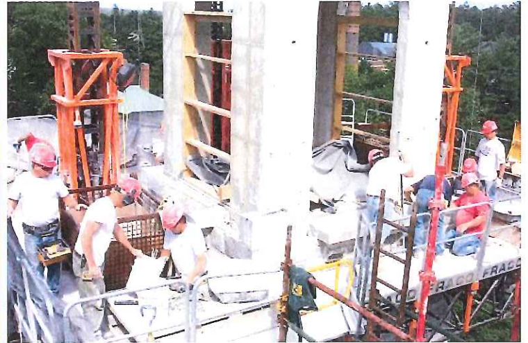
Reconstruction of Backup Wall – using Precast
