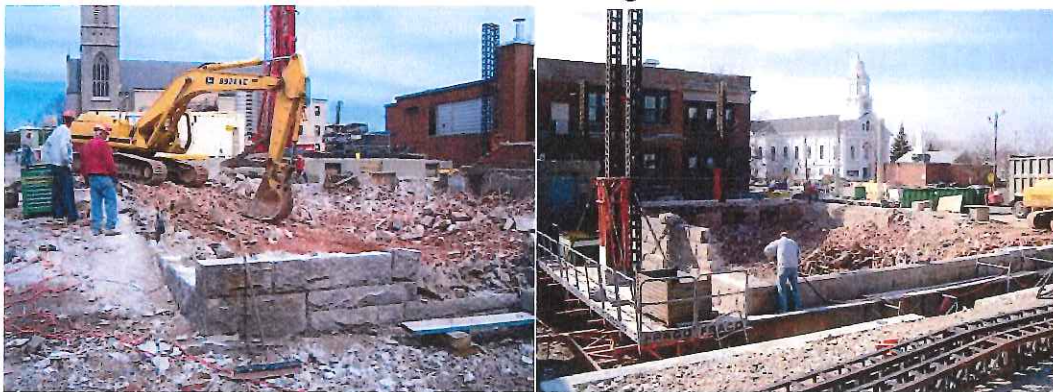
Salvaging Stone Veneer – Demolishing Backup wall Masonry
