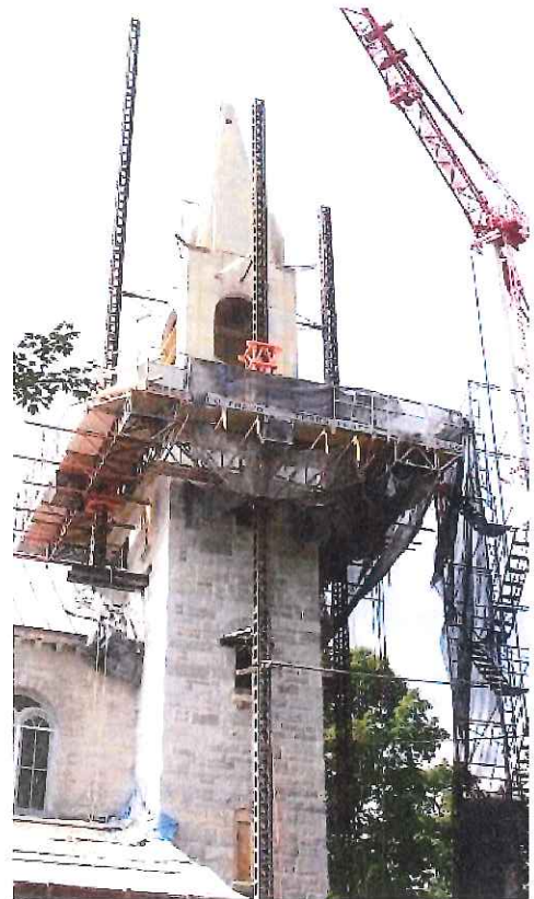
Veneer Reconstruction At Spires Bell Towers - Complete Disassembly and Backup Reconstruction
