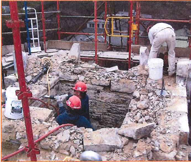
Disassembly of Veneer and Backup Wall
