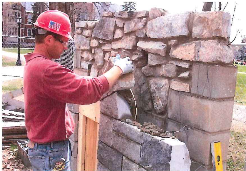
Preconstruction Mockups for Quality Control of coursing
