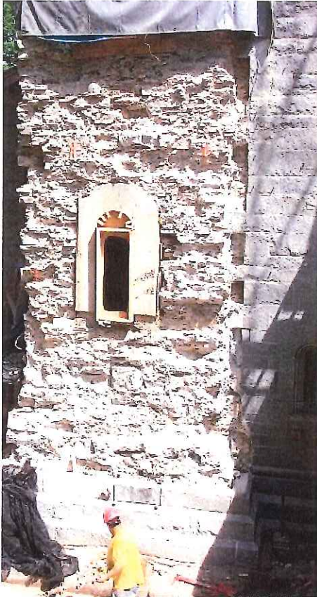
Disassembly of Lower Tower – Veneer Only
