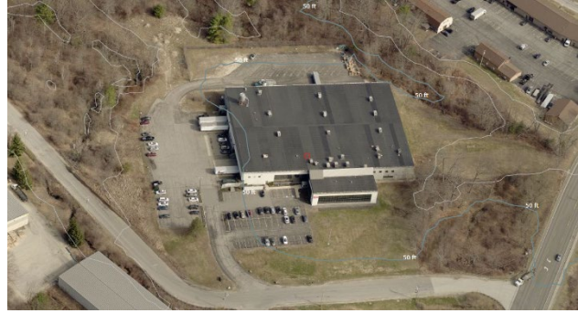
Figure 3. Current Site Conditions
