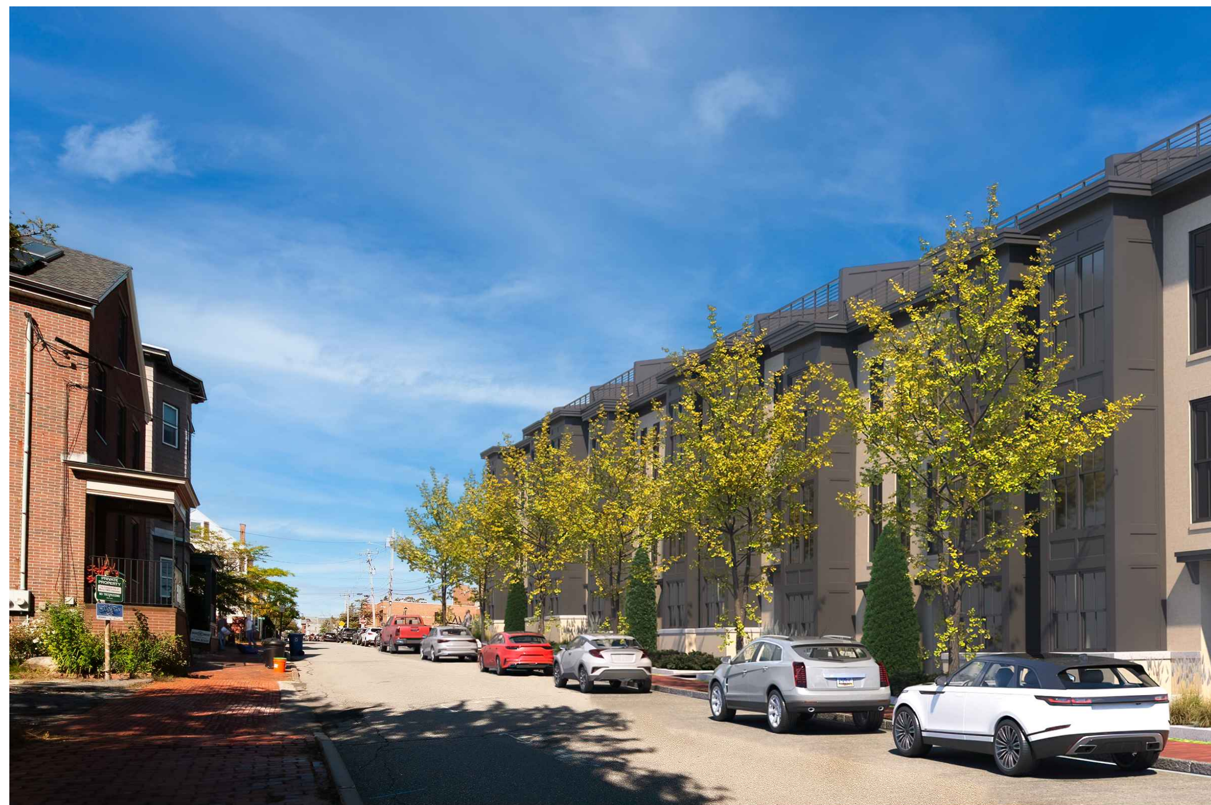
3 VIEW FROM DOWN WINTER STREET
