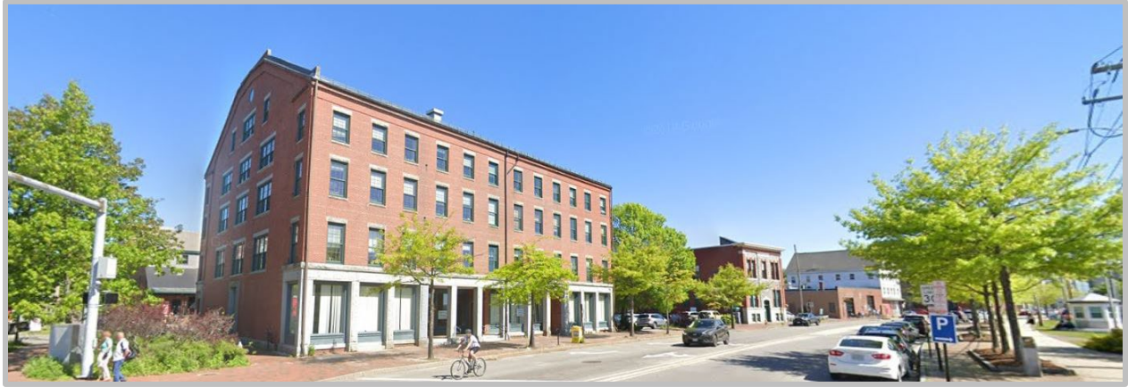
Figure 2: Street View of Commercial Street
