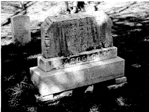
Marble marker with exposed foundation
