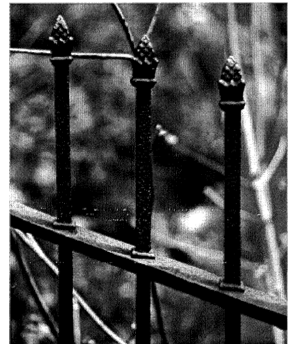
Iron fence at northwest corner
