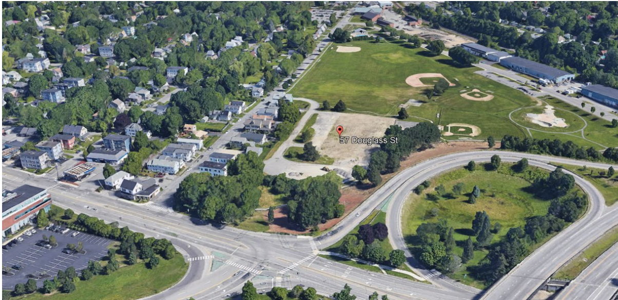
Figure 2: Aerial View of Site (facing north)
