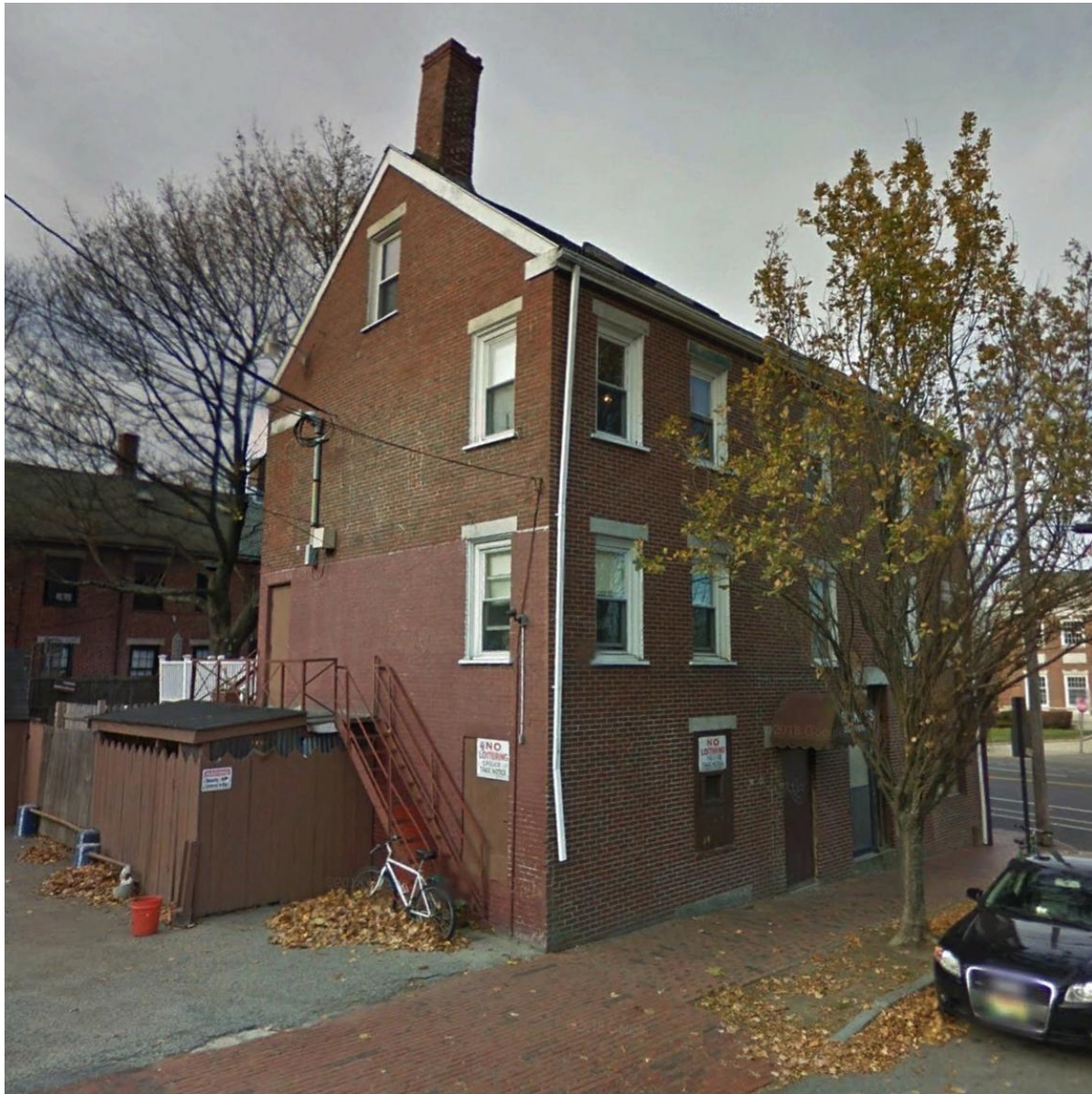
EXISTING BUILDING FROM MECHANIC STREET
