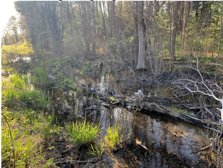
Drainage/Pooling Along Road – May 12, 2020
