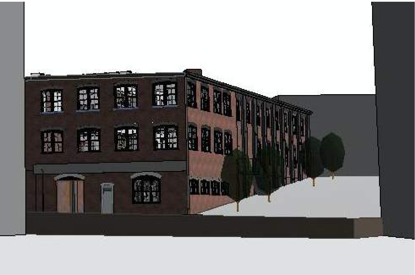
2 VIEW W FROM COMMERCIAL STREET (OUTSIDE HISTORIC DIST.)
