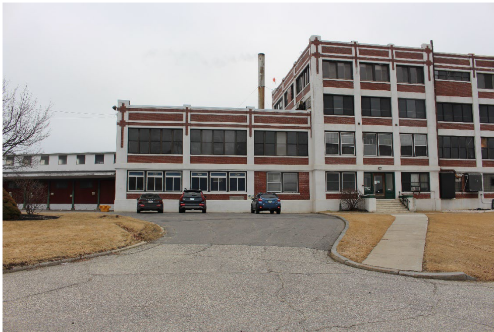
2. B&M Factory, West Elevation, looking east.
