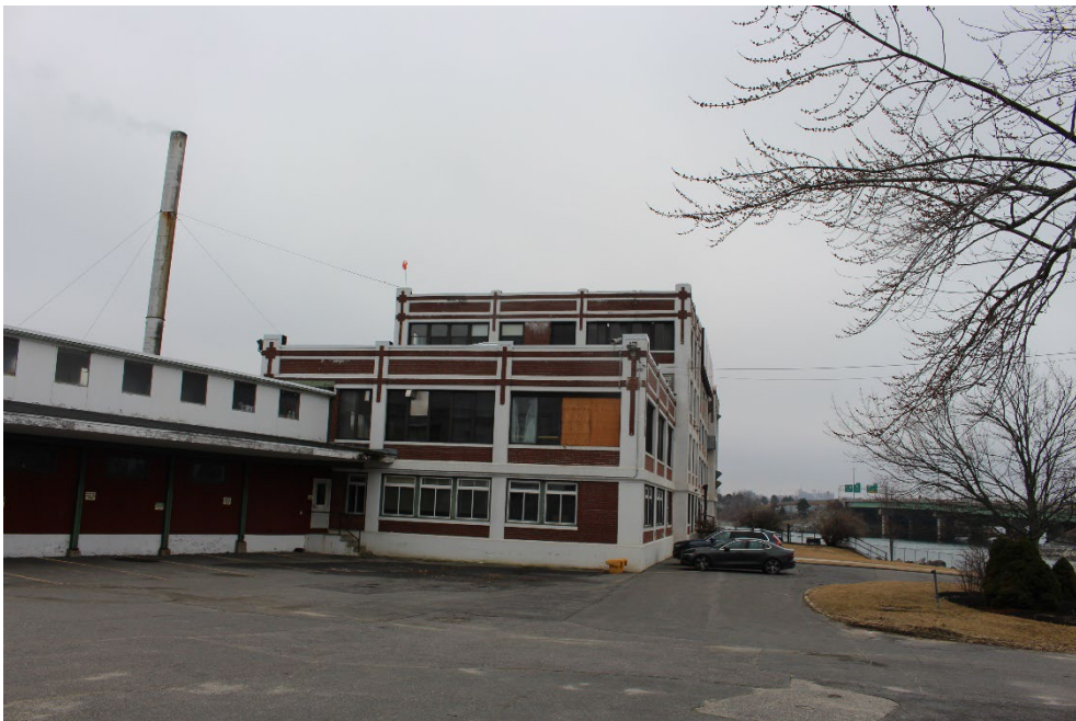
4. B&M Factory, North Elevation, looking south.
