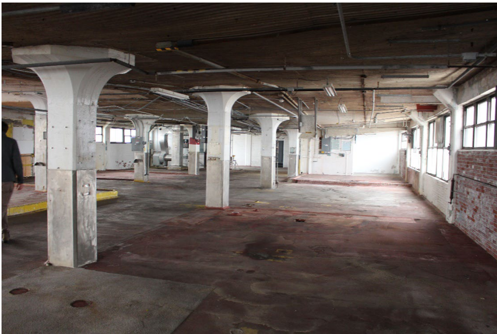
10. B&M Factory, Fourth Floor, looking south.
