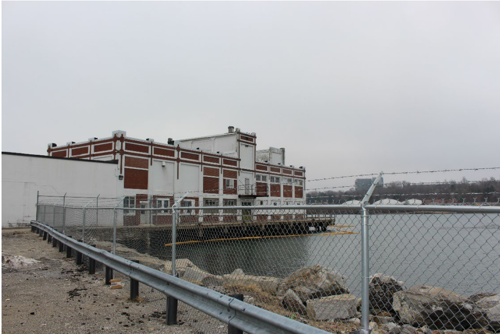
11. Site, Codfish Canning Building, looking southeast.
