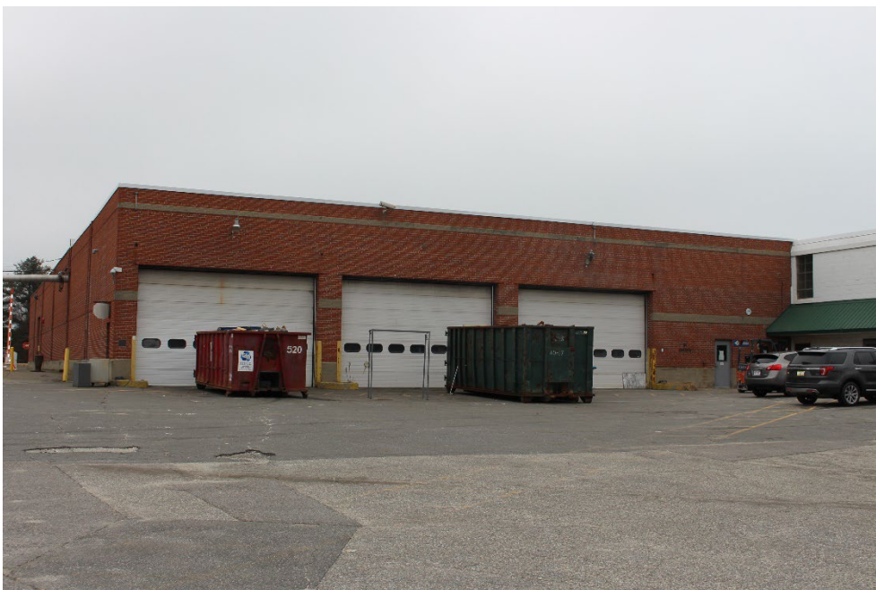
14. Site, Storage/Labeling Building looking northwest.
