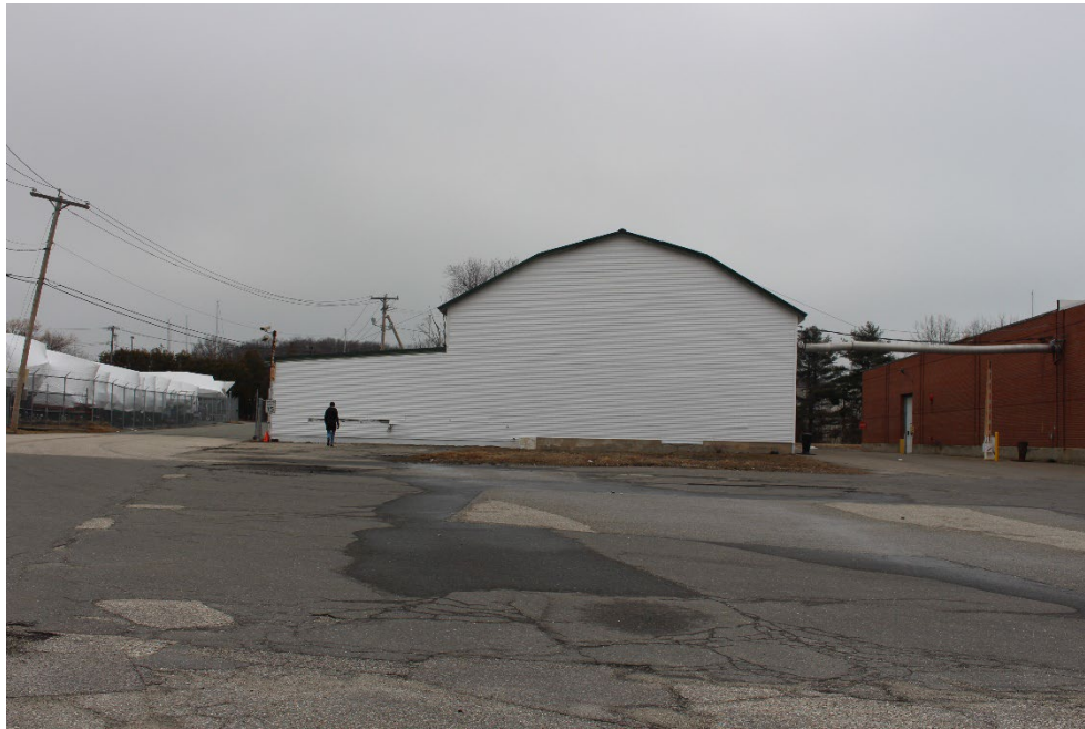
15. Site, Woodworking/Storage Building, looking northwest.
