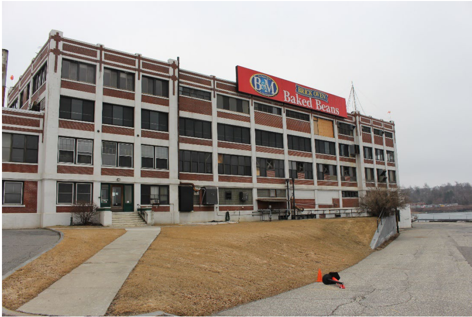
1. B&M Factory, West Elevation, looking southeast.
