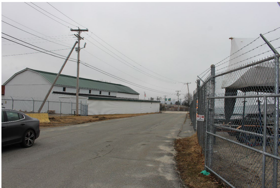
16. Site, Entrance and Woodworking/Storage Building looking south.
