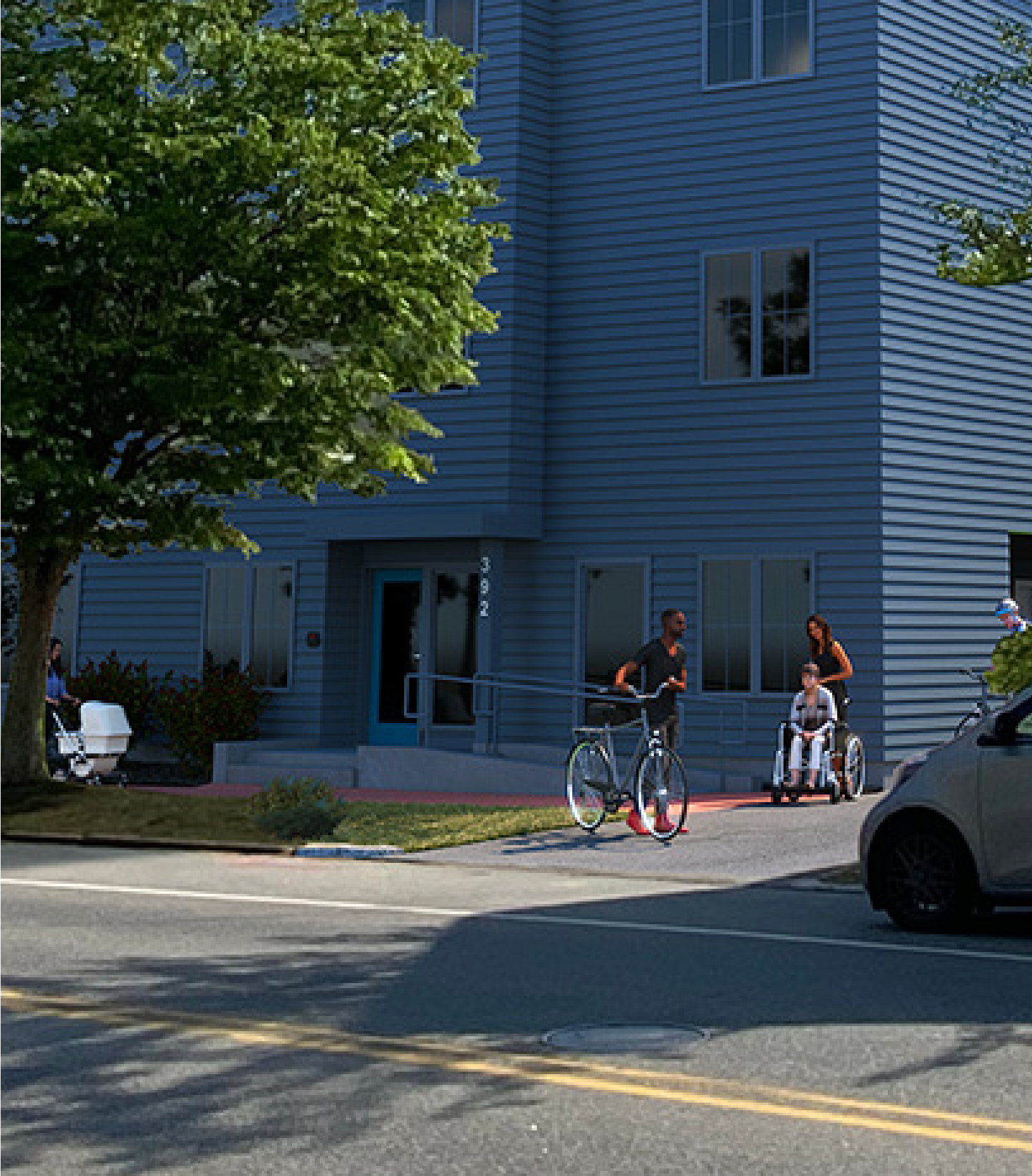
Closeup of ADA ramp, entrance porch and shared driveway.
