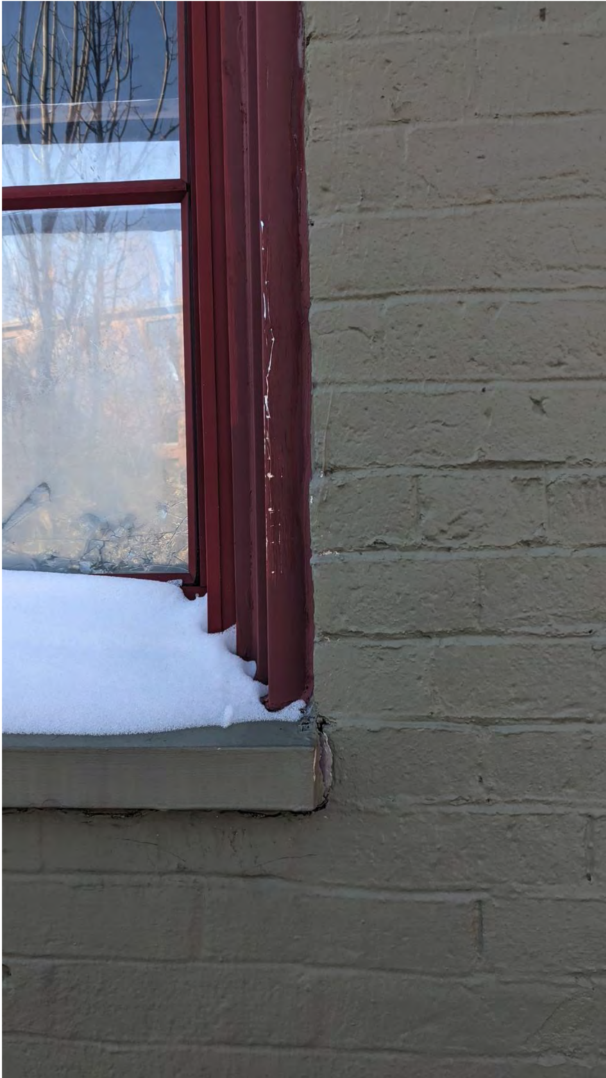
PAINTED BRICK DETAIL
