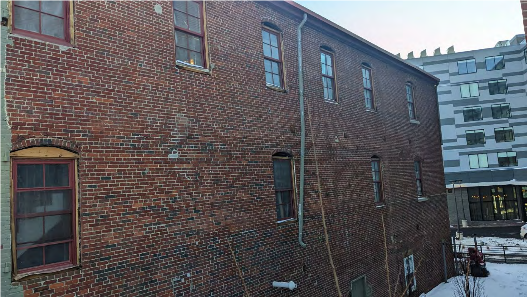
CLEANED BRICK FACADE
