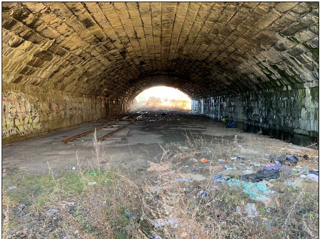
Photo 4 – Existing Railroad Tunnel Under York Street
