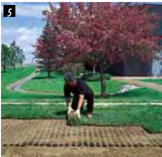
Hydroseed or lay sod.
