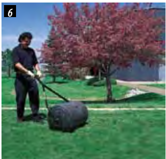
Roll sod with heavy roller.
