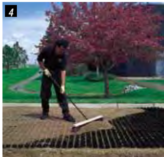
Fill rings with clean sharp concrete sand.
