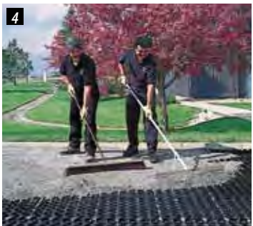
Fill rings with clean gravel.
