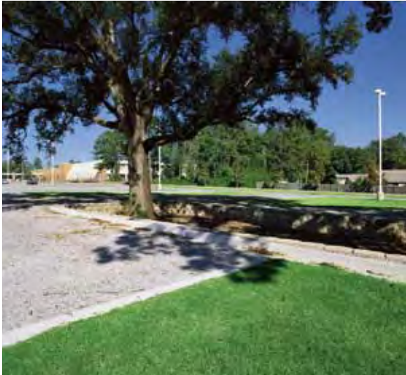
The University of South Alabama, Mobile used Gravelpave 2 in parking aisles and Grasspave 2 in the spaces.
