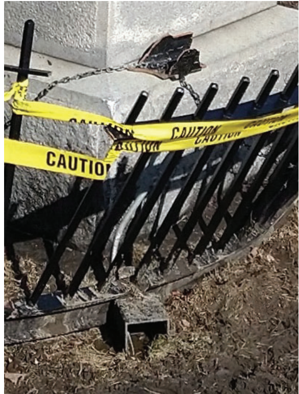
Bollard after accident in 2022
