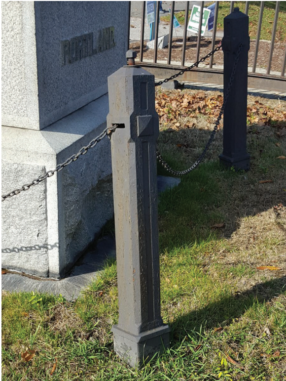
Bollard prior to treatment in 2000
